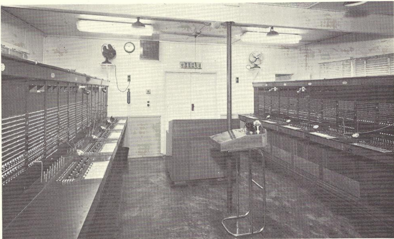
Fig. 1-6 — Large Manual Exchange.
