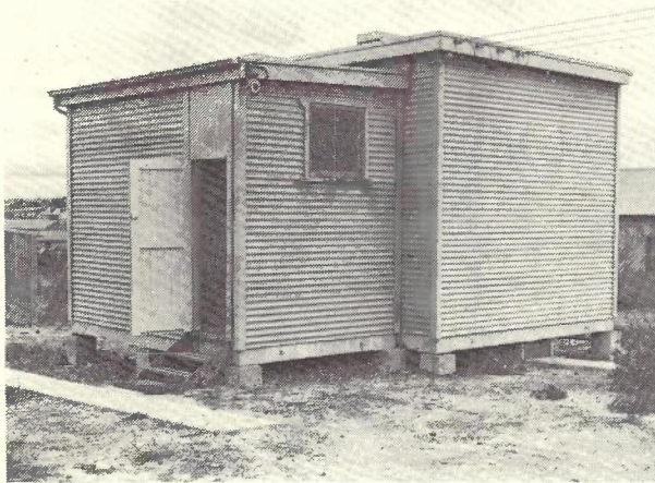
Fig. 1-7 — Transportable Telephone Exchange.
