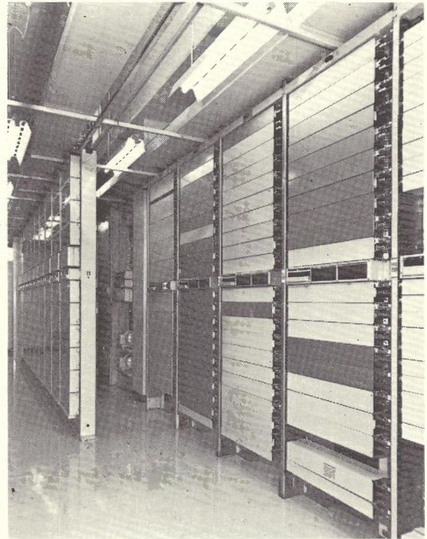
Fig. 1-8 — Crossbar Exchange Racks.
