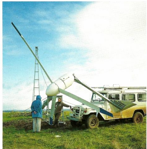
Telecom Australia is already the worlds biggest user of photovoltaic (solar module) technology. TRL is now researching the use of hybrid solar/wind energy systems to power repeater stations in remote locations
