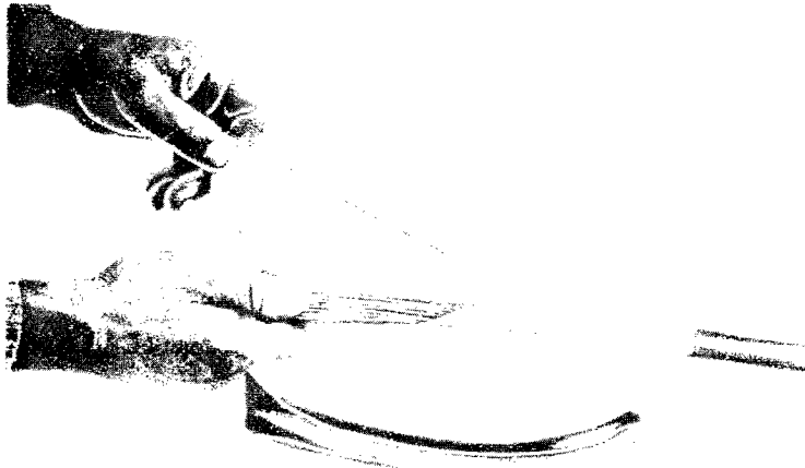
FIG. 17. PEEL OFF REST OF LEAD.
