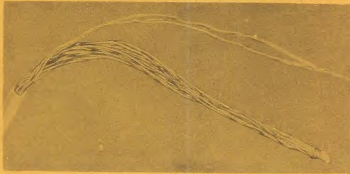
FIG. 5. BUTTED CABLE READY FOR FANNING.
