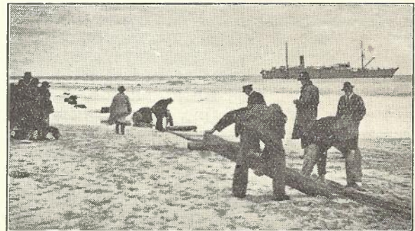
Fig. 1. Hauling end of cable ashore at Apollo Bay, using float barrels every 10 fathoms.
