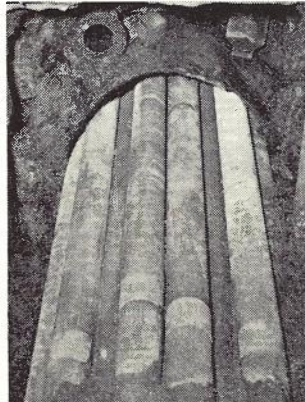
Fig. 1.—The pipes at one end of the main. Part of this particular section was in open trench. Note the flush-fitting collars.
