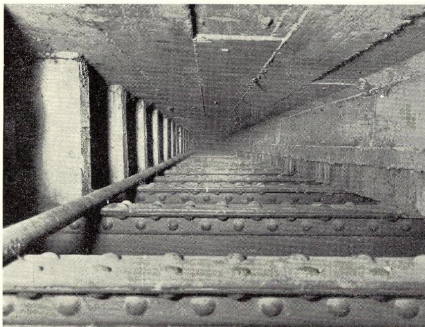
Fig. 3.—View beneath footway on main spans before installation of pipes.
