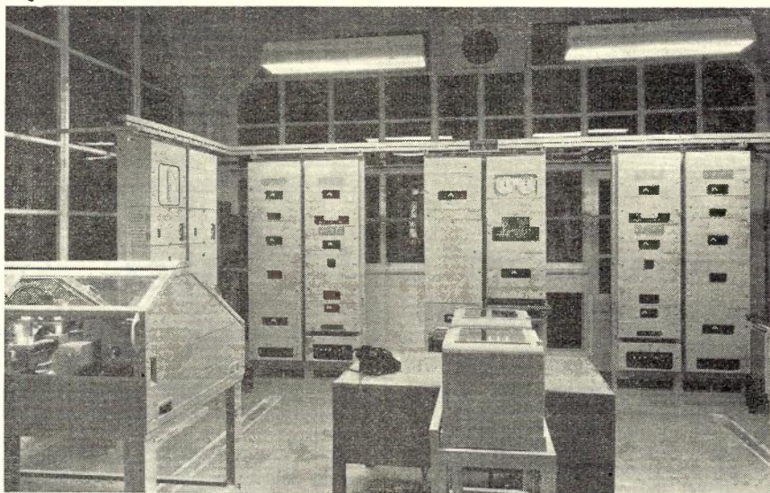
Fig. 2.—Speaking clock installation 1st floor City West Exchange, Melbourne.
