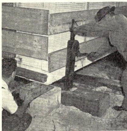
Fig. 6.—Jacking up Exchange.
