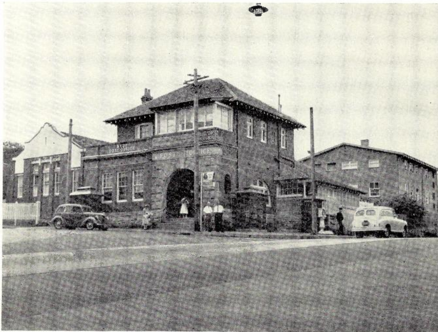
Fig. 3.—Ryde Post Office and Exchange Buildings Today.
