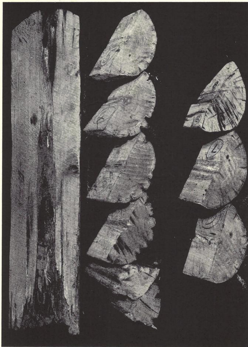
Fig. 1.—Butt (4' long) section of Red Stringybark, ( E. Macrorrhyncha ) pole erected 1931, taken from Willow Tree—Tamworth Section. Extensive internal rot of fungal origin tapering into the central region towards upper end. Extension of the rot above ground, by way of the central pipe, would be quite probable, especially in damp situations. No insect damage visible.
