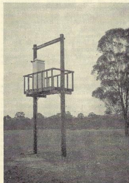
Fig. 5.—Pole Mounted Repeater Marsden Park.
