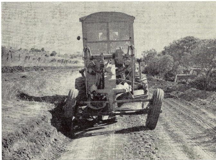
Fig. 10.—Grader Excavating beside Cable, under control of the Locator.
