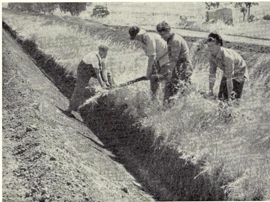
Fig. 17.—Placing the Cable in the new trench. (Following operations shown in Fig. 16).
