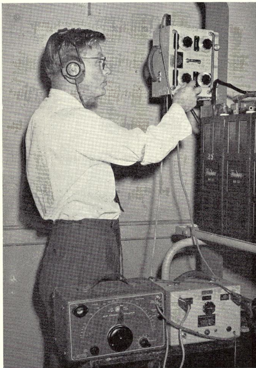
Fig. 5.—Busbar Impedance Bridge and Tuned Detector in Use.
