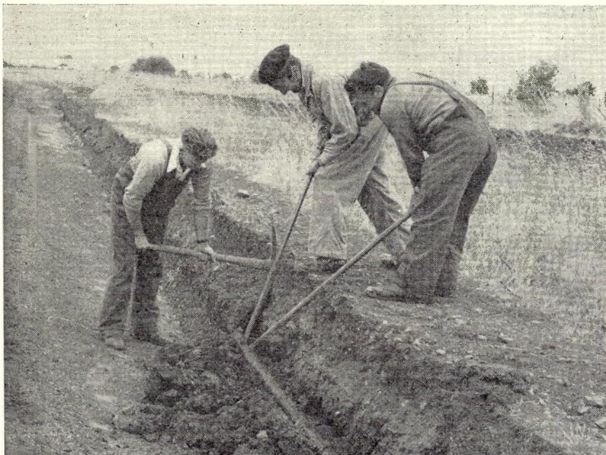
Fig. 16.—Removing Cable from the side of the Trench following mechanical excavation by Grader.
