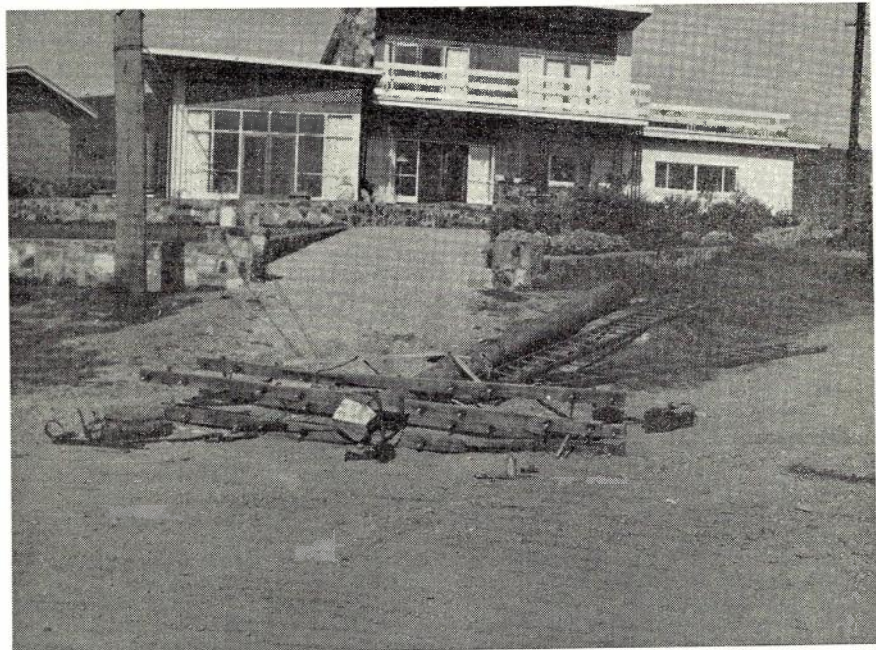
Fig. 1.—This condemned pole fell whilst two linemen were at work on it removing spindles and insulators. The hazard could have been eliminated by dropping the pole to the ground complete with fittings.
