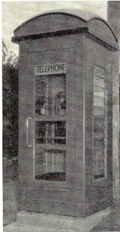
Fig. 5.—Louvre-Glazed Wooden Cabinet.
