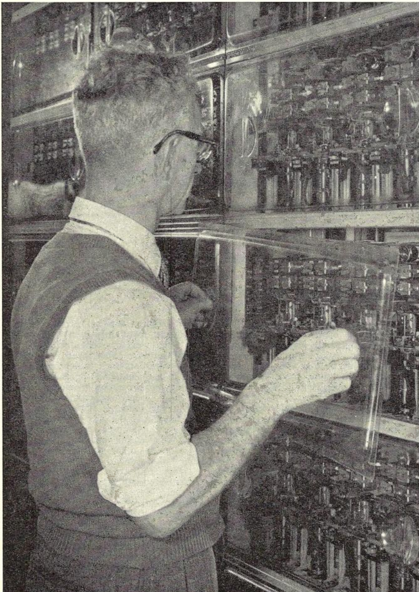
Fig. 8.—The author removes a panel. Vertical bars are also removable.
