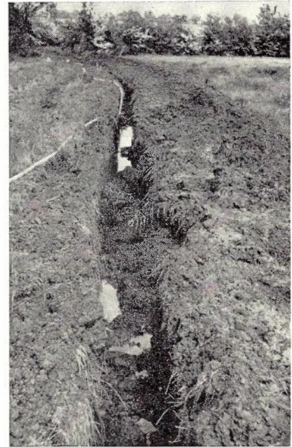
Fig. 10.—Example of trench collapse.
