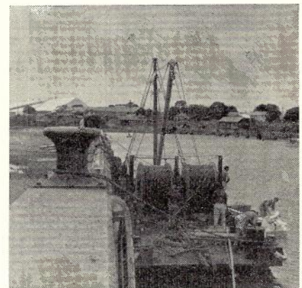
Fig. 3.—Front view of barge showing: 1.—lay-out of supports. 2.—Guying arrangement. 3.—Fair Lead, Main Cable Brake and Bow Sheaves. Cable was fed from drum, through Fair Lead, Brake, Bow Sheaves round the prow of the barge and under the barge.
