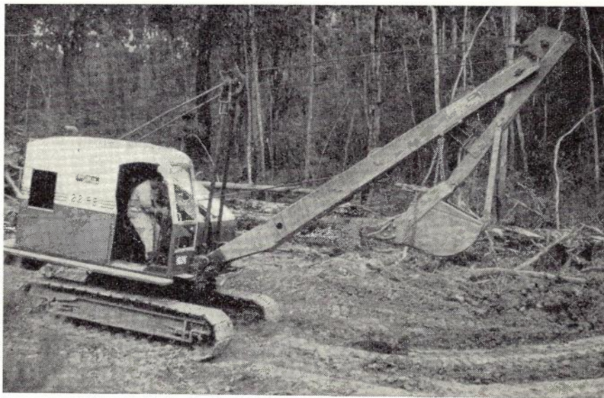
Fig. 5.—22RB Excavator rigged as Backacter.
