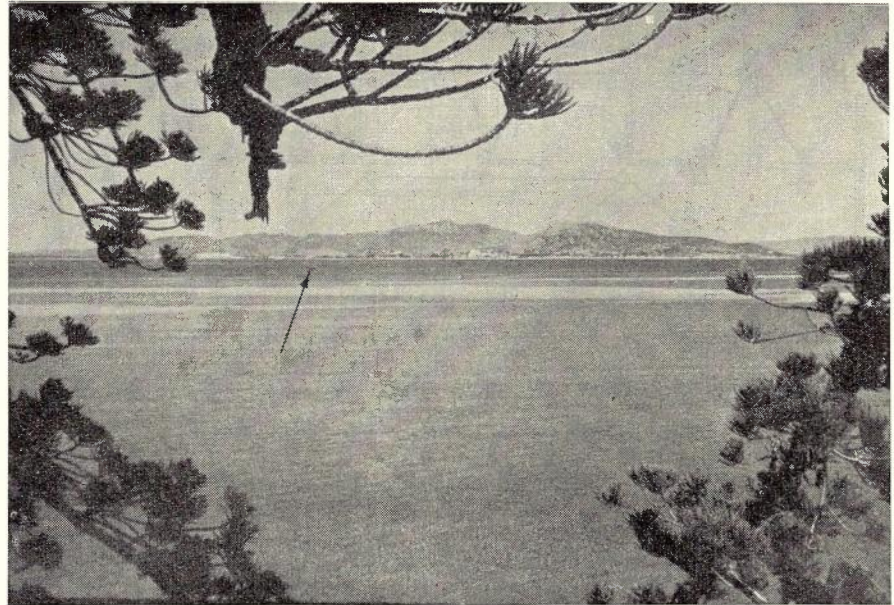
Fig. 1.—A view of the 5½ miles cable route looking from Magnetic Island towards Townsville. The pontoon indicated by the arrow may be observed working at No. 8 joint.
