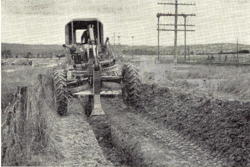
Fig. 15.—Grader consolidating back fill. Note front wheels off ground.
