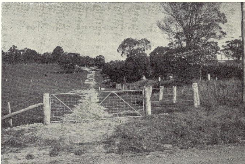
Fig. 1.—Gate installed on the cable route by the gate party.
