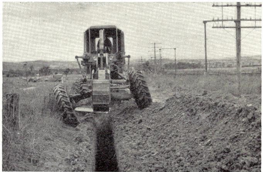
Fig. 14.—Grader backfilling trench.
