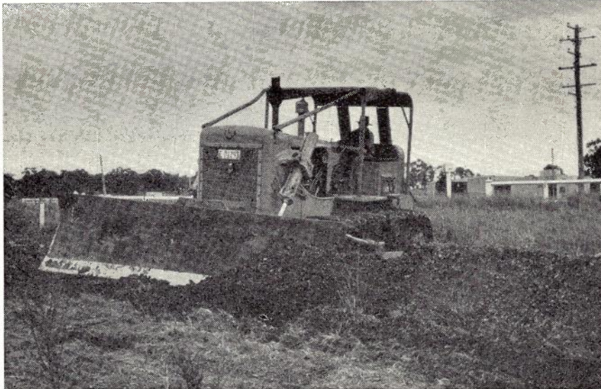
Fig. 13.—H.D.16 Tractor backfilling trench.
