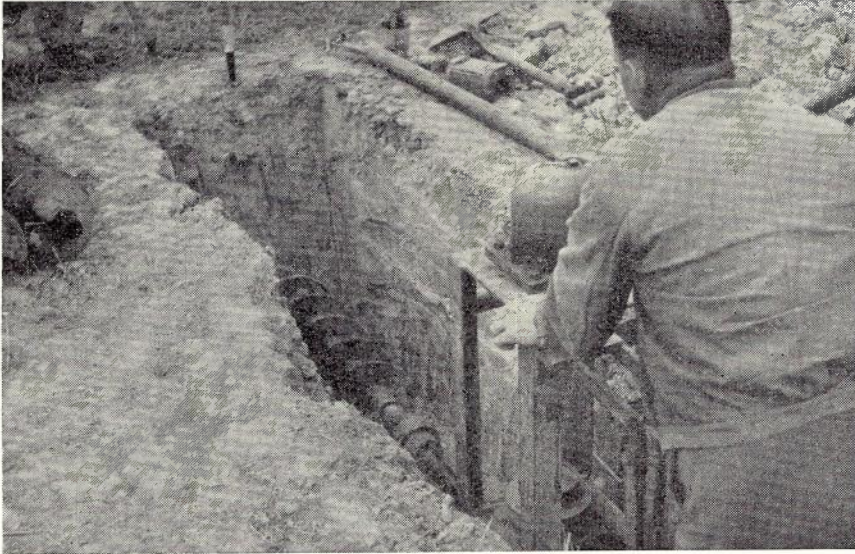
Fig. 3.—Proline Horizontal Borer showing Auger.
