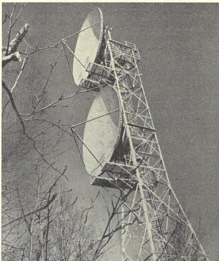
Over-horizon radio relay system (spanning more than 125 miles) for 120 telephone channels per radio frequency.
