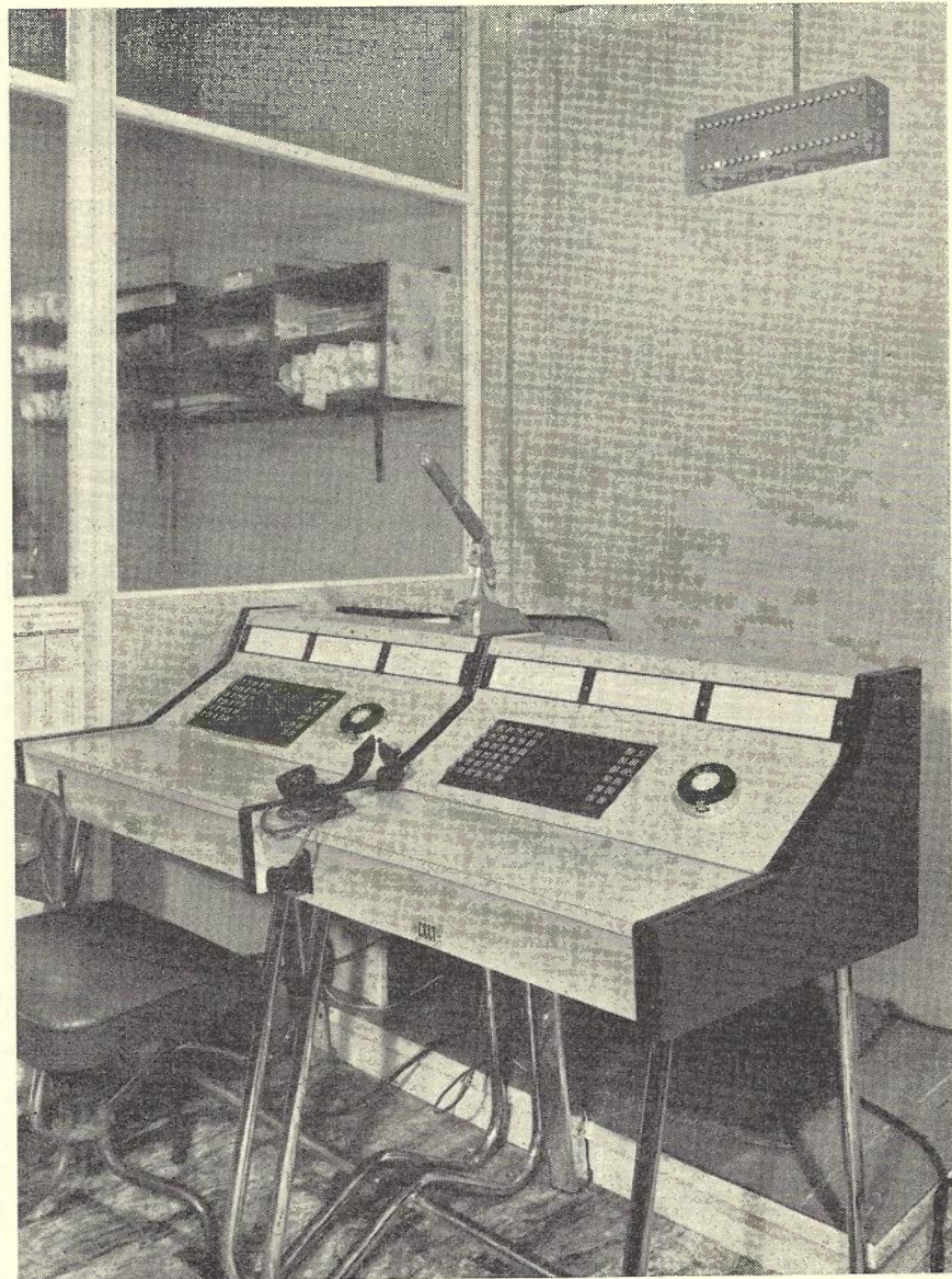
Fig. 8.—Operators positions, showing on the wall the exchange line indicating lamp strip.
