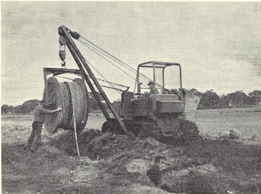
Fig. 20.—Laying Cable with HD.11 Side Boom Crane.
