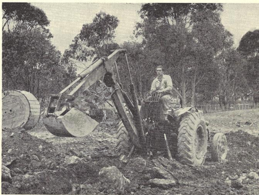
Fig. 8.—Ace Back Hoe Excavating Trench in Rocky Ground After Ripping.
