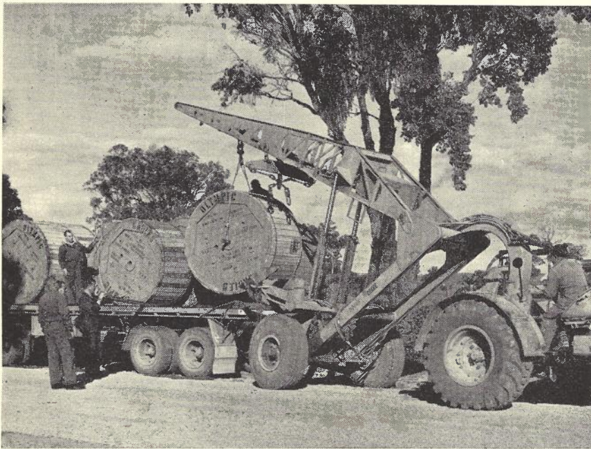
Fig. 2.—Unloading Vehicles in the Field.
