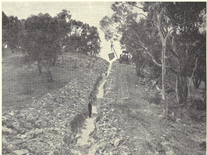
Fig. 19.—Depositing Bedding Sand from Hopper on HD.11 Side Boom Crane.
