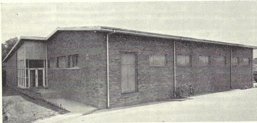
Fig. 2.—Campbelltown Communication Building.
