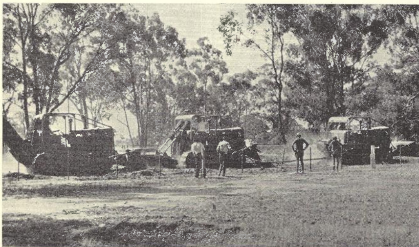
Fig. 14.—Tandem Ripping, one HD. 16 Tractor pushing and one HD. 16 Tractor pulling the Ripping Tractor.
