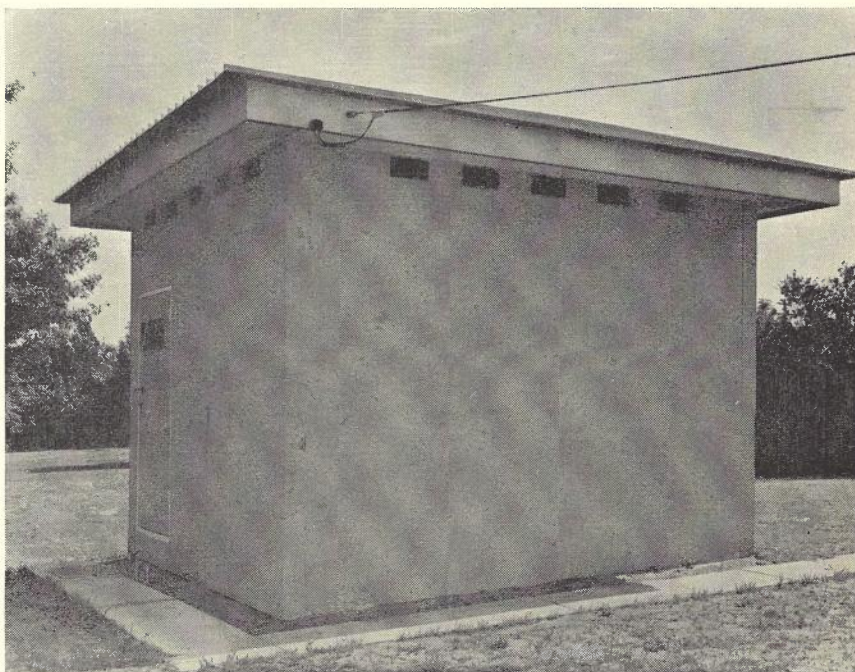
Fig. 1.—Typical Unattended Repeater Building.
