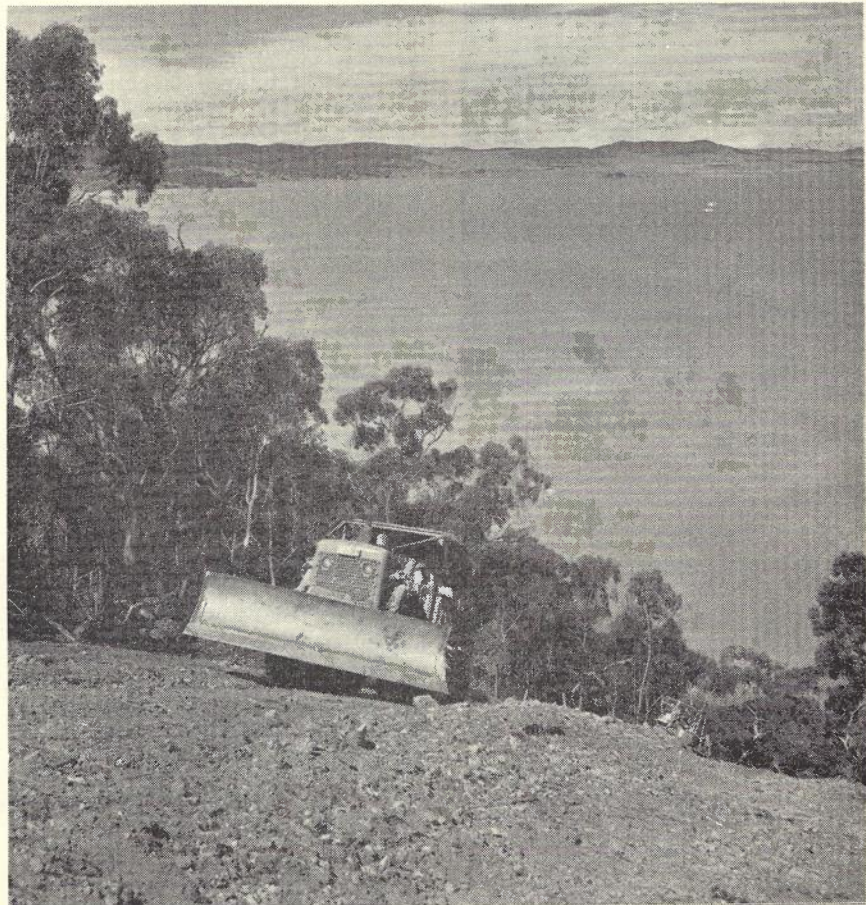
Fig. 22.—Backfilling Trench on Escarpment at Lake George near Canberra. O.C.12 Tractor which is Backfilling the Trench is Anchored by the Winch Rope of the HD.16 Tractor in the Foreground.
