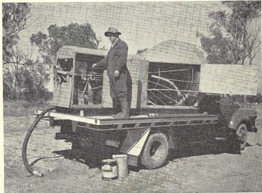
Fig. 32.—Roductor Duct Rodding Machine.
