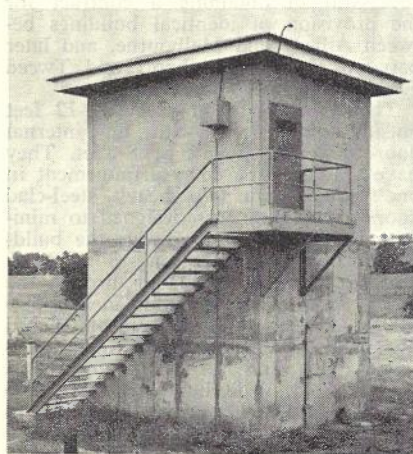
Fig. 5.—Unattended Building in Area Subject to Flooding.
