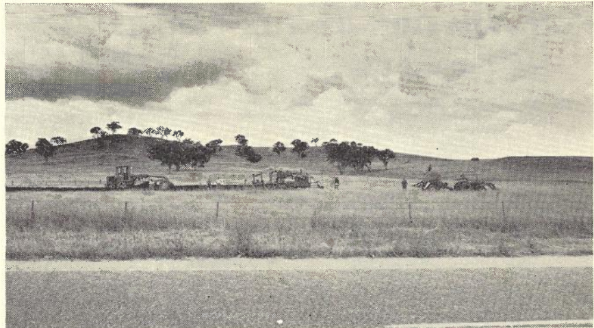
Fig. 4.—Cable Laying and Backfilling.
