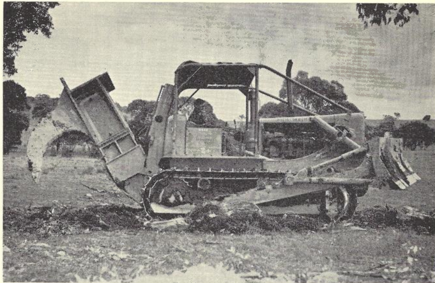
Fig. 13.—HD. 16 Tractor with 4 ft. Ripper Tine.
