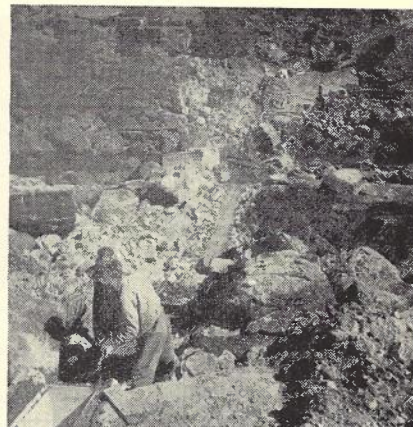
Fig. 27.—Laying Polythene Pipes Under Nepean River Crossing at Pheasant's Nest Pass near Campbelltown.
