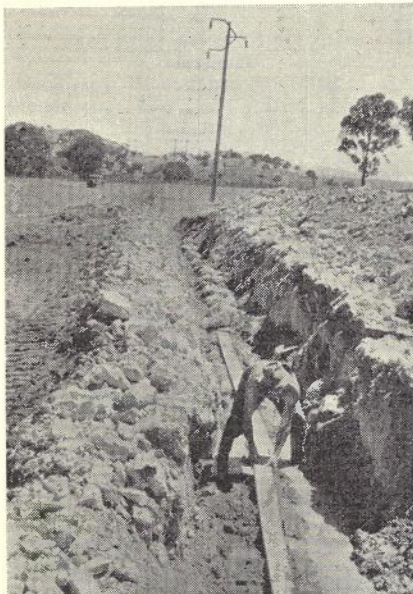
Fig. 21.—Placing Planks on Overbedding Sand in Rock Trench.
