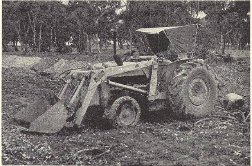
Fig. 24.—Tractor Mounted Compressor and Front End Loader.
