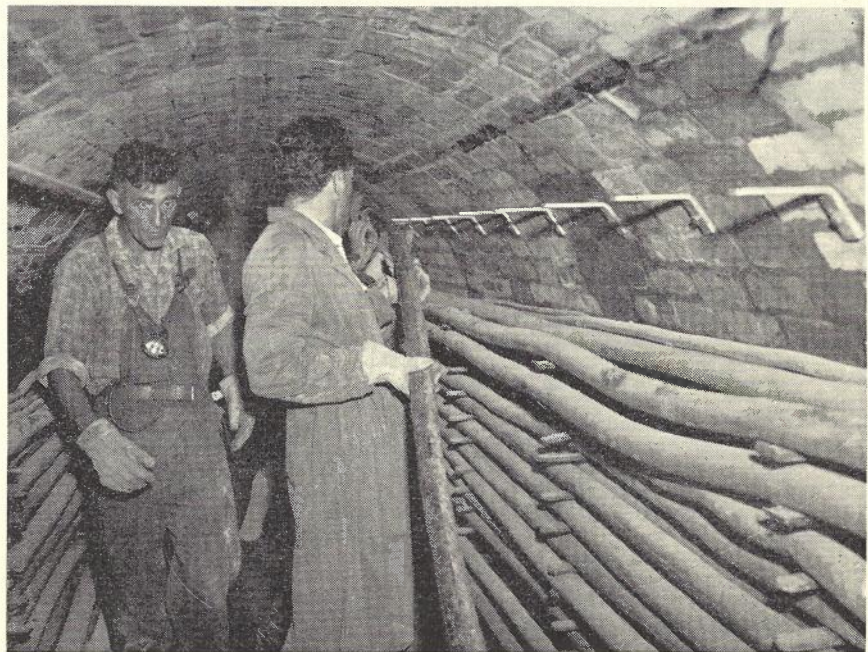
Fig. 30.—Laying the First Length of Cable in the Tunnel from Terminal at Sydney.
