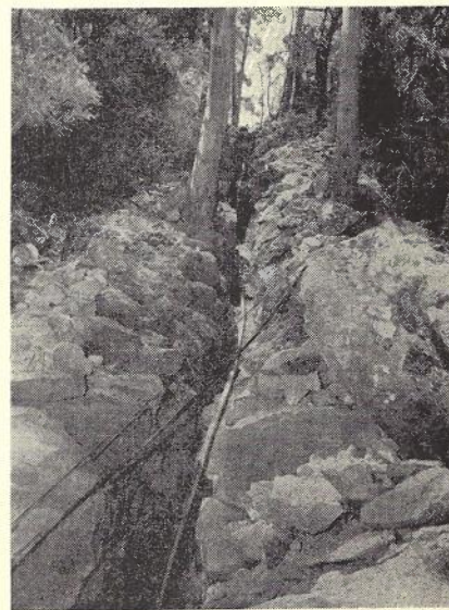
Fig. 28.—Trench on the Approach to the Nepean River Crossing at Douglas Park near Campbelltown.
