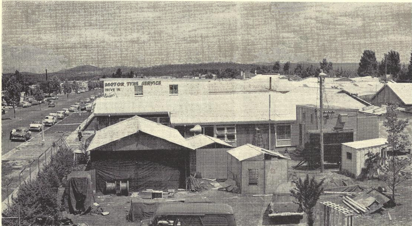
Fig. 7.—General View of Civic Site on 30/10/1961. Line Depot Building is in Centre Left with Extensions Complete, Temporary Installation Store is in Bottom Left, with Ironworkers Shop adjacent. Portable Exchanges are in Centre Foreground.
