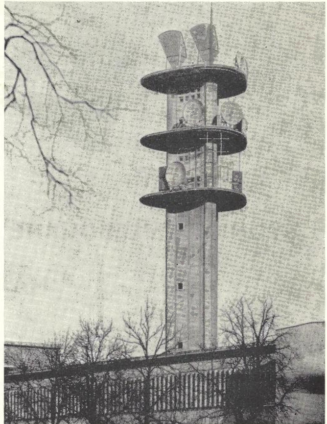
Communication tower of a large station
