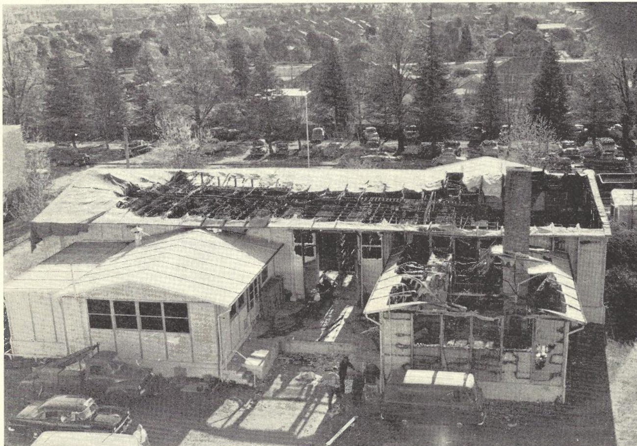
Fig. 1.—Looking down on Damaged Building, showing Destruction of Air Treatment and Equipment Areas.
