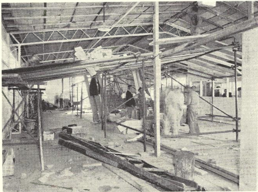
Fig. 6.—Scene inside the Line Depot Building on the Day of the Fire. New M.D.F. is being Erected and Roof Insulation is in Progress.
