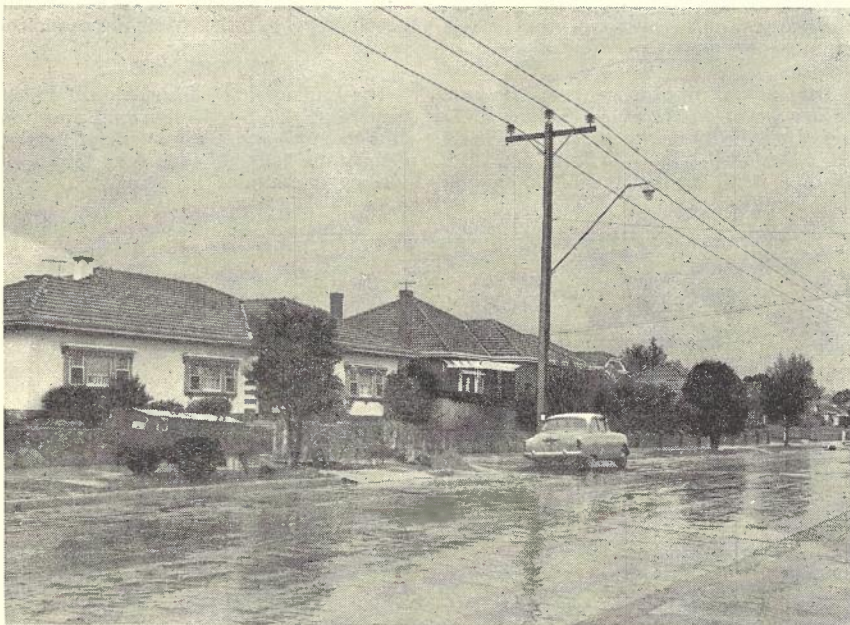
Fig. 2.—66 kV Line in Poath Road.
