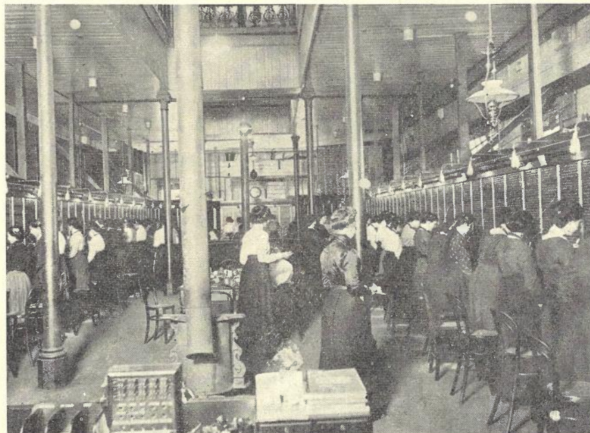
Fig. 7.—Main Switchroom, First Floor, Central Telephone Exchange, Wills Street, 1908.
