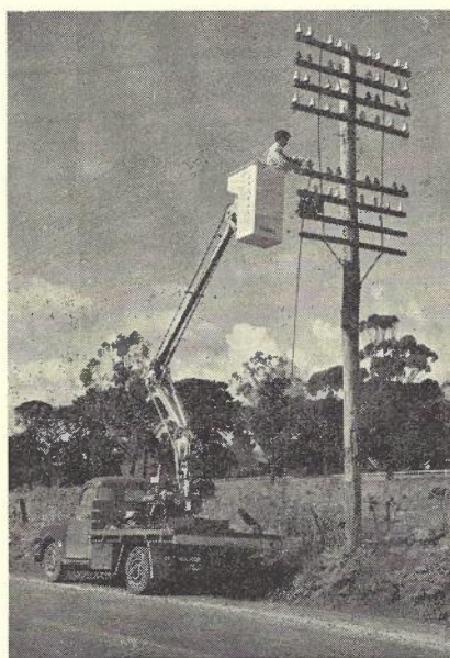
Fig. 1.—(b) Hydraulic work platform.
