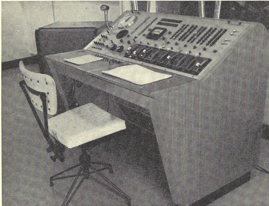
Fig. 4.—Continuity Suite Desk Equipment. Control Booth Operator's Desk.
