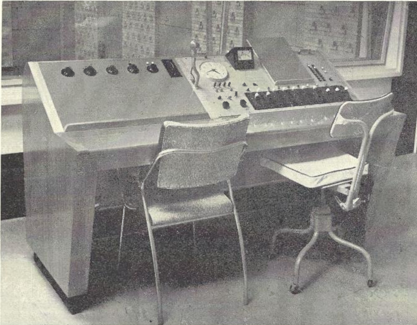
Fig. 9.—Production Studio Control Desk. Showing Facilities for Operator and Producer.
