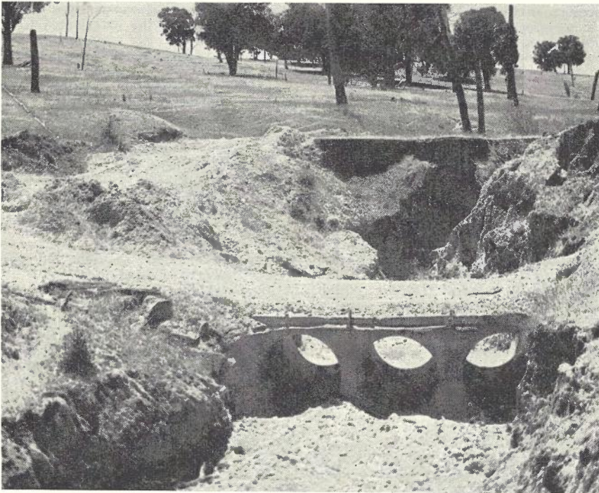
Fig. 2.—Patrol Access Track Crossing Soil Erosion Gully. Cable is buried through this crossing.
