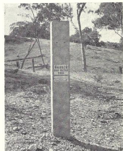
Fig. 3.—Typical Cable Marker Post Erected in Cross-country Section.
