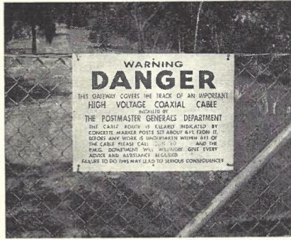
Fig. 4. — Warning Sign on Access Gateway. Buried cable passes through such gates erected on property boundaries.
