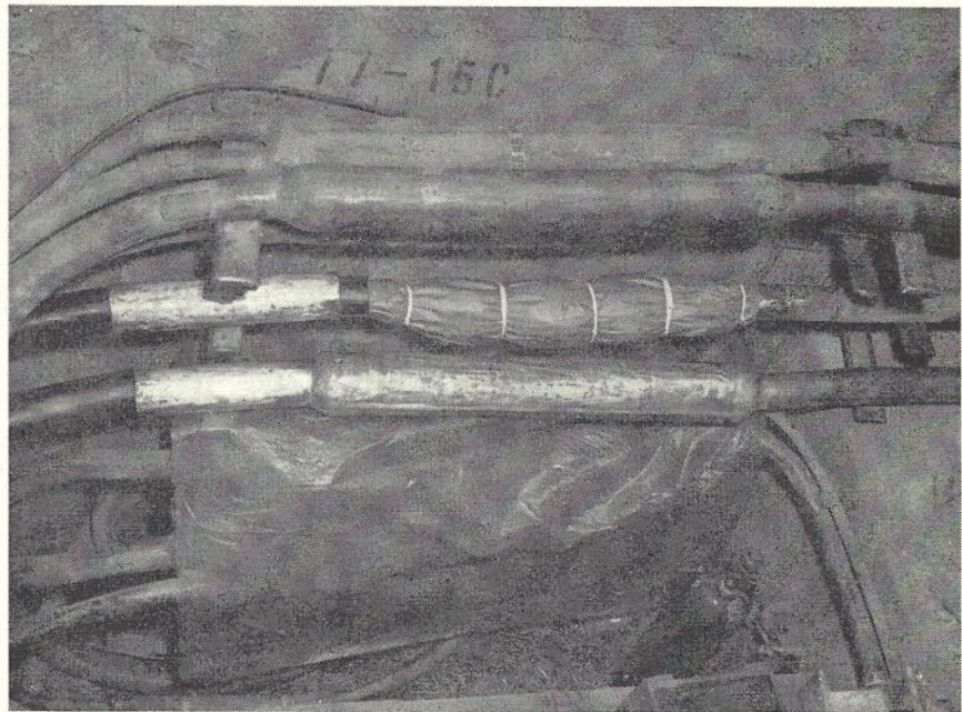
Fig. 3.—Plastic-lead Joint in Manhole. In the upper joint, the auxiliary sleeve is in place and the main sleeve has yet to be fitted; the lower joint is completed.
