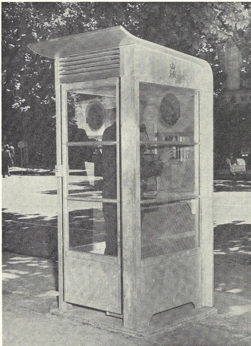
Fig. 8.—Aluminium Public Telephone Cabinet.
