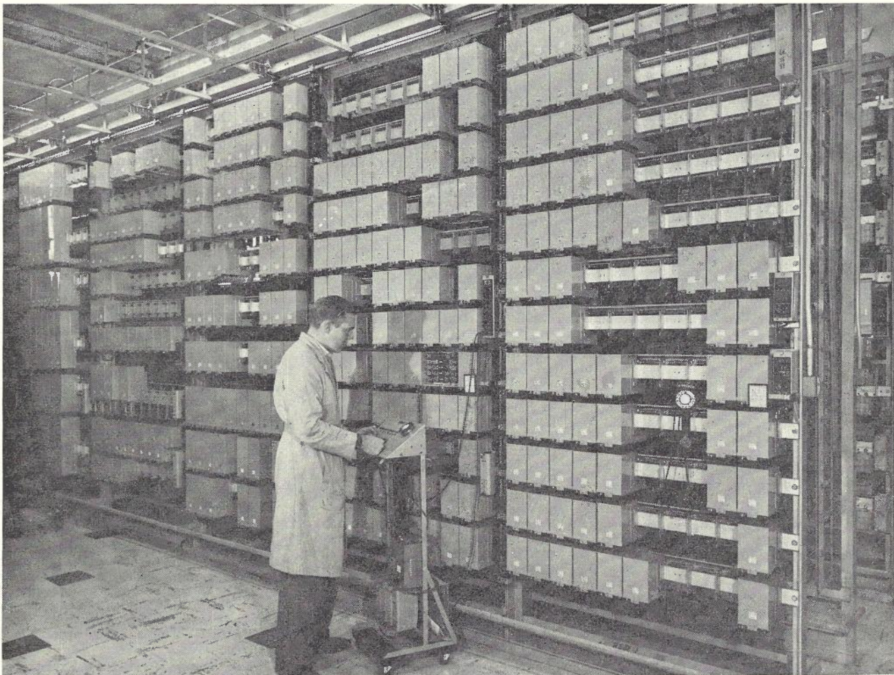
Fig. 2.—2,000 Type Equipment Racks.
