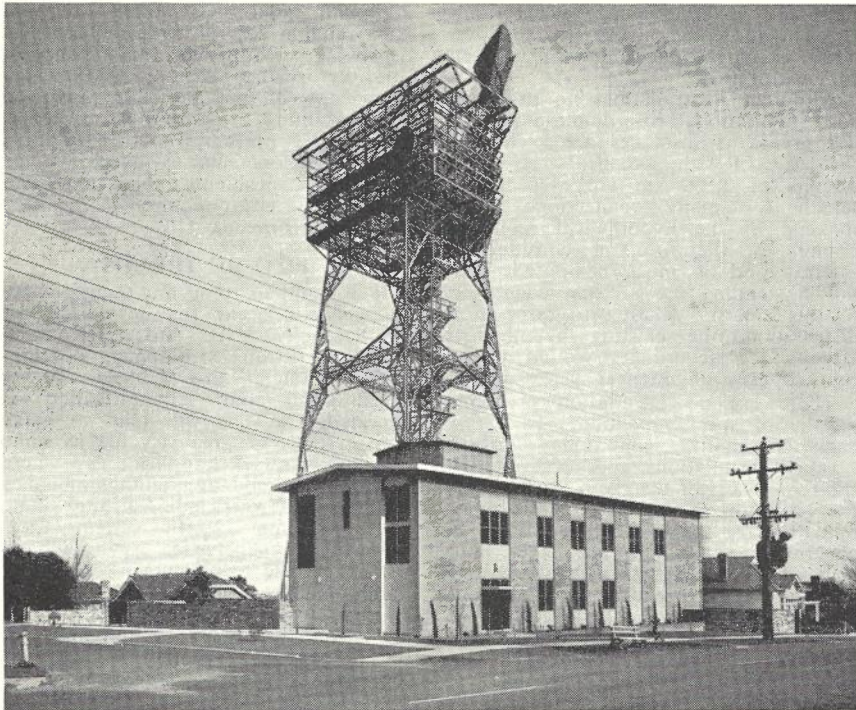
Fig. 3.—A Modern Radio Terminal Established in a Suburban Location in a Capital City. Provision has been made in the building and aerial support structure for future development and expansion.
