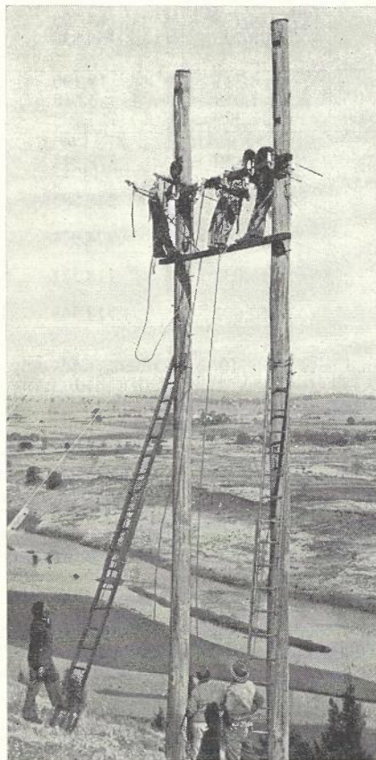
Linemen fit plastic vibration dampers on a 1,600 ft. aerial wire span over the Hunter River, New South Wales, an area of regular floods.
