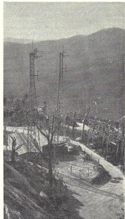
Mt. Oberon (Victoria) station of Victoria-Tasmania Radio Telephone circuit. The station is unattended and generates its own power from diesel engines.
