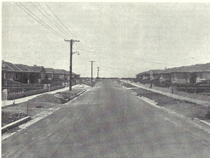
Fig. 6.—Distribution of Telephones to Residential Subscribers by Aerial Drop Lead. Underground plastic distribution cable feeds terminal box on each pole to which drop wire leads are connected. This is joint-use construction; the poles belong to the Power Authority and carry both telephone and power wires. In some cases a separate line of telephone poles is erected along the free side of the street.
