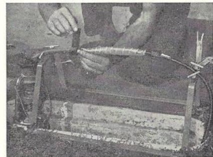
1.—Preparing for lead sleeve.
