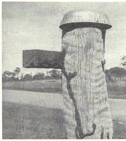
Termite attack on a test pole and crossarm in Northern Queensland—one of a series in a field trial of preservative measures.
