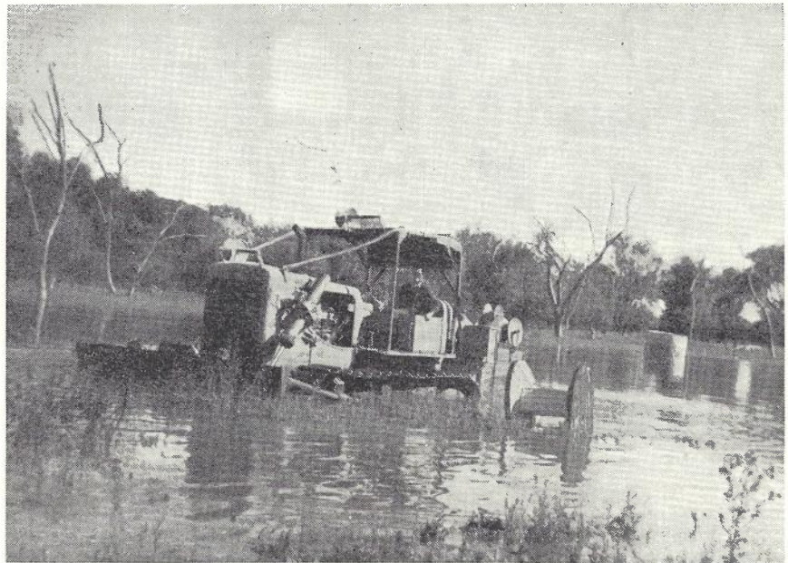
Fig. 5.—Tractor Ploughing Cable in Flooded Country.
