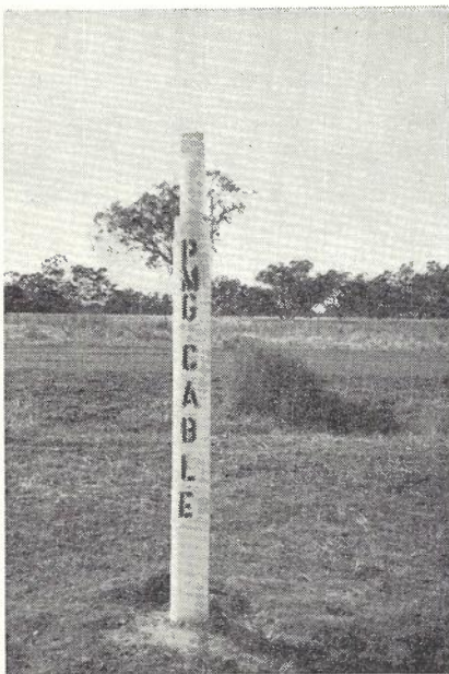
Fig. 7.—Completed Above-ground Joint.
