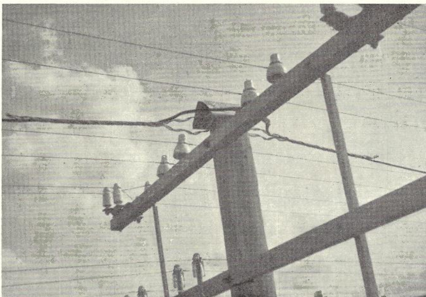
Fig. 2.—Cable Termination at Straight Through Joint.
