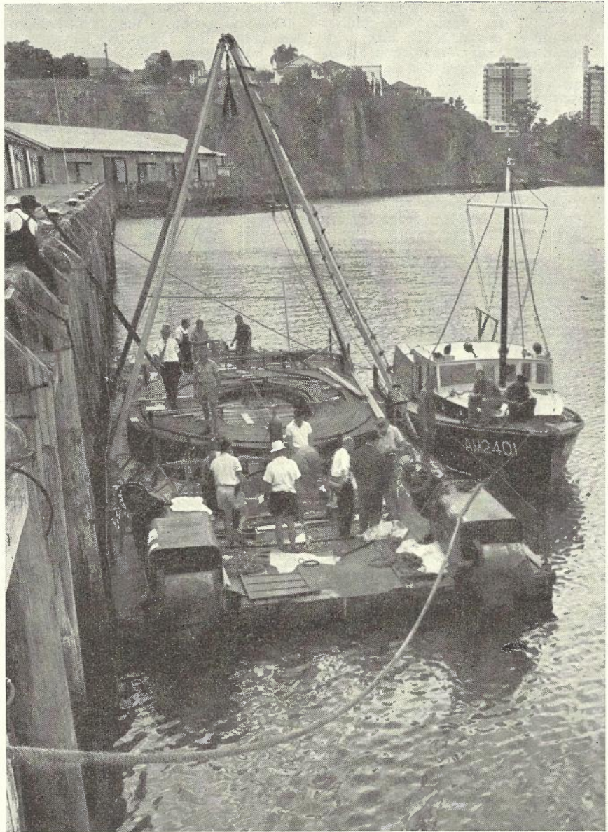
Fig. 4.—Cable Jointing Proceeding on Army Barge N.L.E. Note in foreground two inboard outboard 115 h.p. engines with propellers which can be raised through 180° and rotated through 360°.
