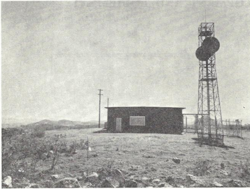
Fig. 3 — Typical Repeater Station.
