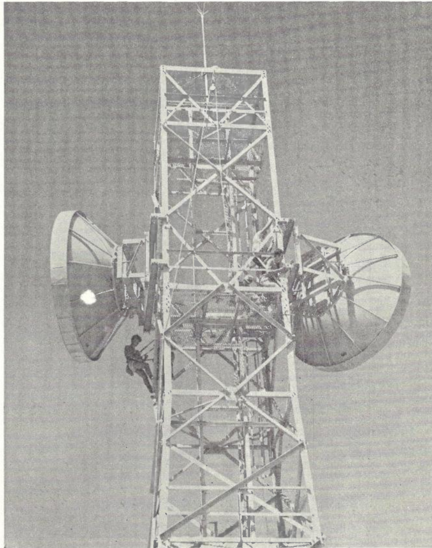
Fig. 6 — Mounting Aerial Systems.
