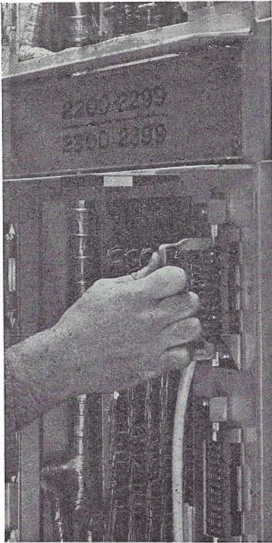
Fig. 6 — An LR/BR Connection Being Fitted.
