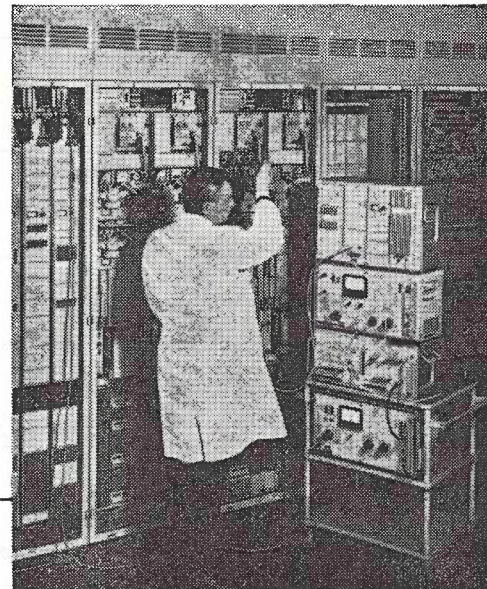
An FM 1800/6000 installation.
