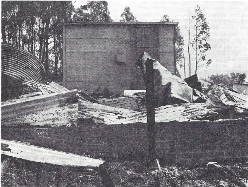
Fig. 5 — Emergency 200 Line Transportable Exchange in Position Adjacent to Completely Destroyed Automatic Exchange at Kettering.
