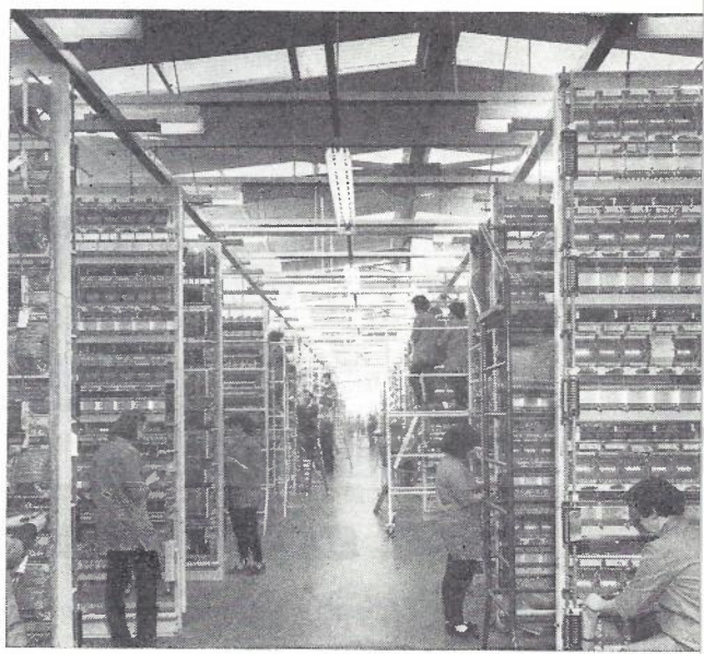
A view of the vast rack wiring sections in the new factory at Kirkcaldy.
