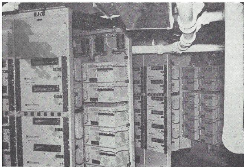
Fig. 7 — A Section of the Tape Recorder Racks.
