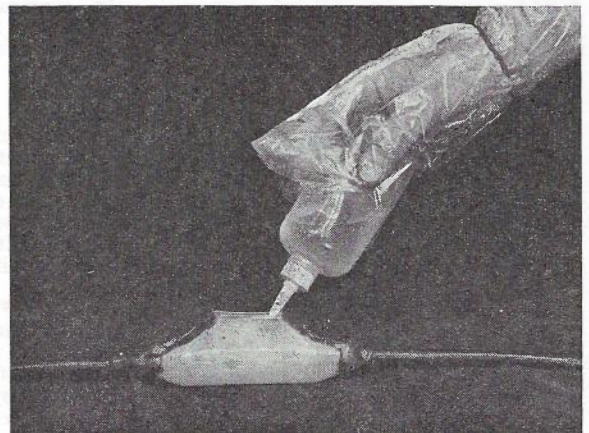
Fig. 17. — Repair Joint in 'Submarine Mould'
