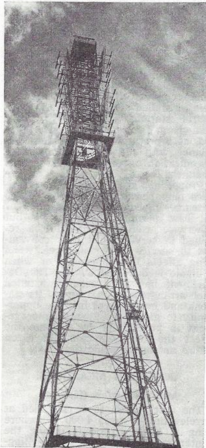
Fig. 12 — Band I Antenna at Mt. Wellington, Hobart, When Panels Were Tilted.
