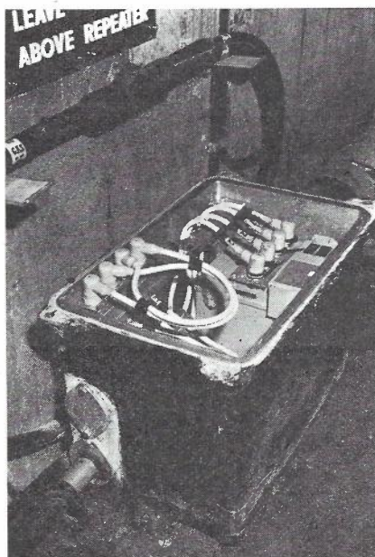
Fig. 15 — Typical A.P.O. Underground Housing with 4MHz Repeater installed and Spare Coaxial Tubes Patched Through.
