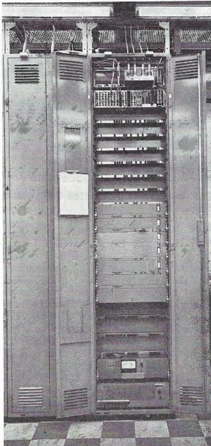
Fig. 17 — Line Amplifier Rack for Terminal and Main Repeater Stations.
