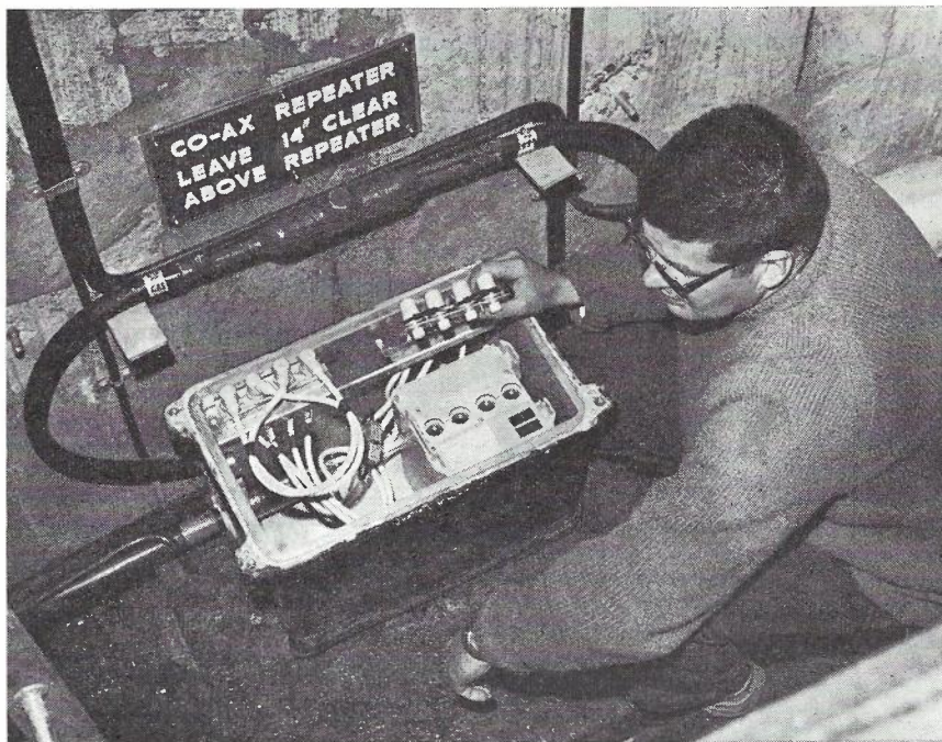
Fig. 16 — Coaxial Cable Pothead Terminations About to be Connected to Repeater Input Sockets.
