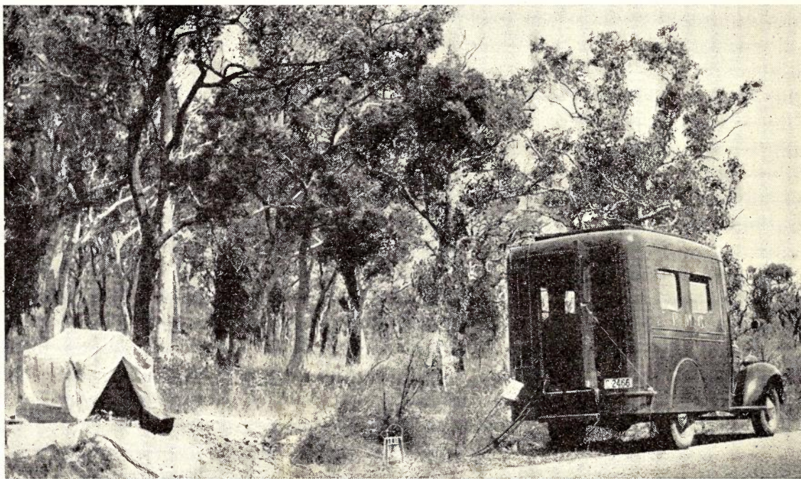
Fig. 3.—Test Van on the Work.
