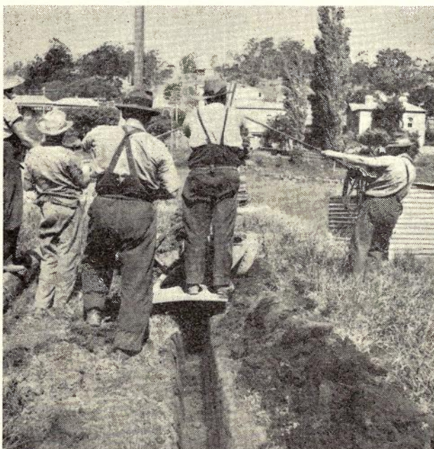
Fig. 7.—Trenching Plough in use near Gosford.
