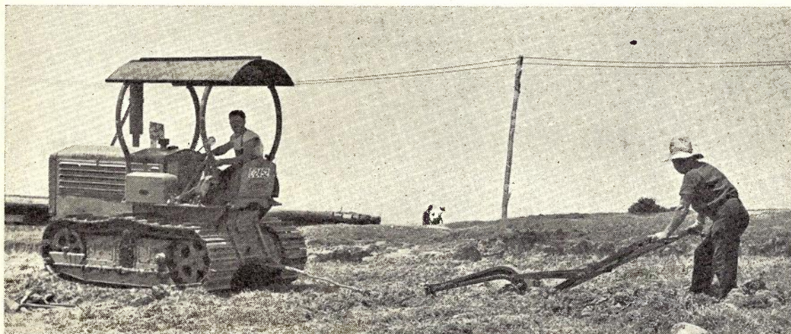
Fig. 6.—Preliminary Ploughing prior to Cable Laying by Mole Plough.
