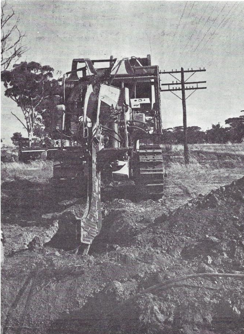
Fig. 4. — A Rear View of the Cable Layer Illustrating Shute and Cable Box Detail.
