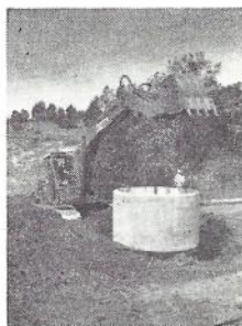
COVER Installing the Perth-Carnarvon Cable
