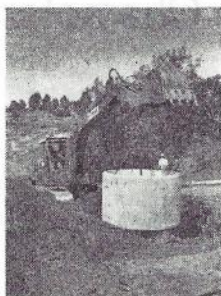
COVER Installing the Perth-Carnarvon Cable
