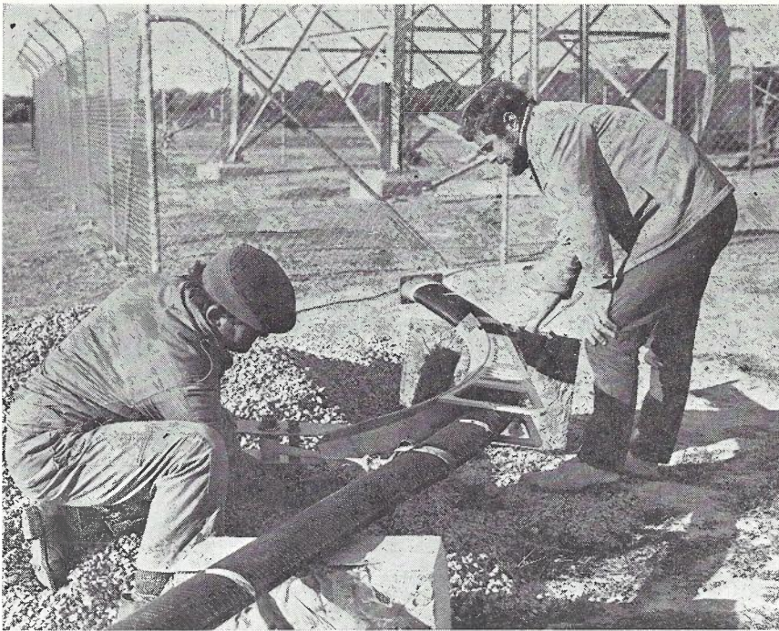
Fig. 2. — Preparation of H-Plane Bend Using Special Bending Tool.
