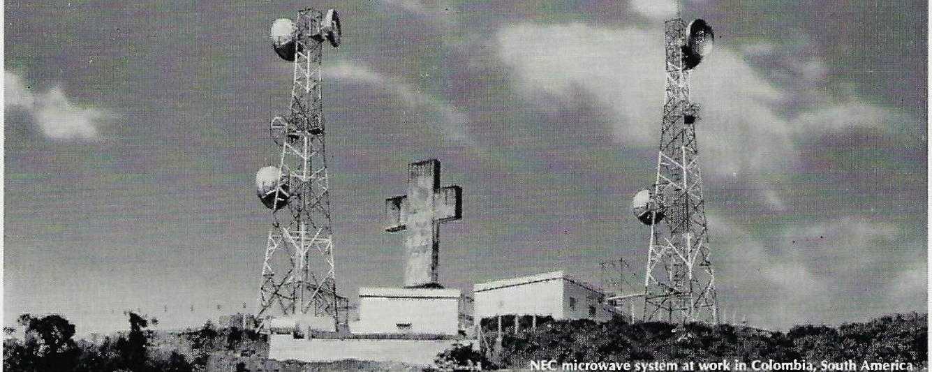
NEC microwave system at work in Colombia, South America
