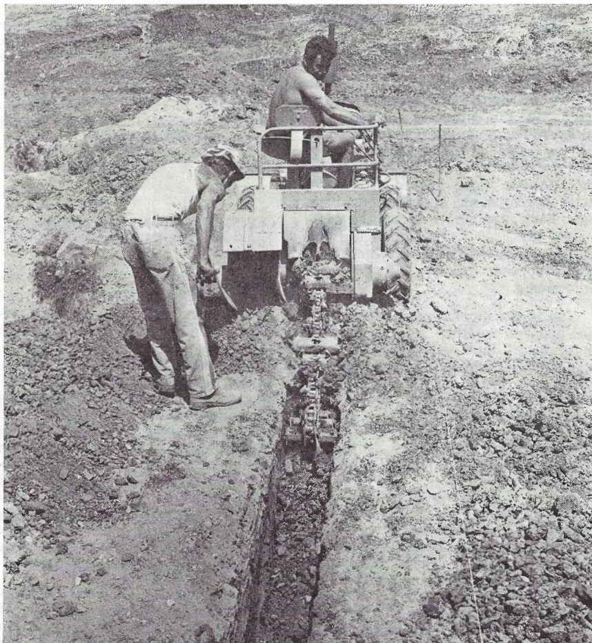
Fig. 3 — Trenching for Cables.
