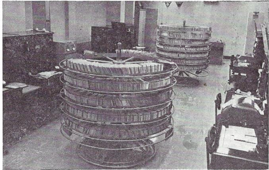
Fig. 5 — Plant Layout — The Two Modules of Edison F.D.C. — Capacity 60,000 Telephone Stations per Module.
