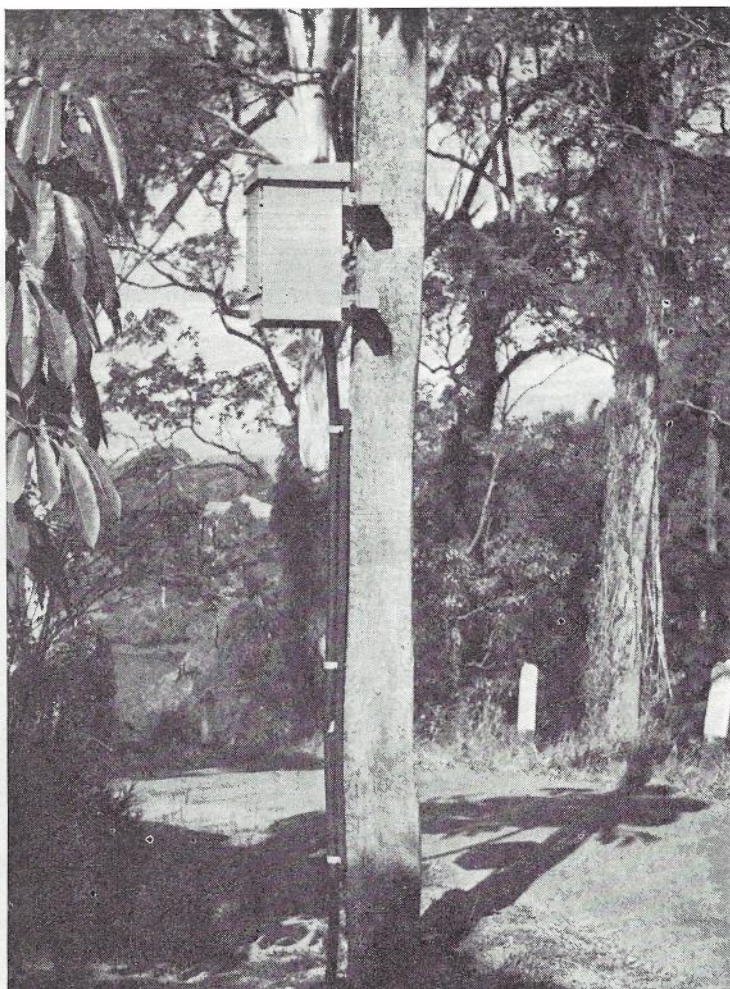
Fig. 5 — Pole Mounted 0.5 kW Cathodic Protection Rectifier.
