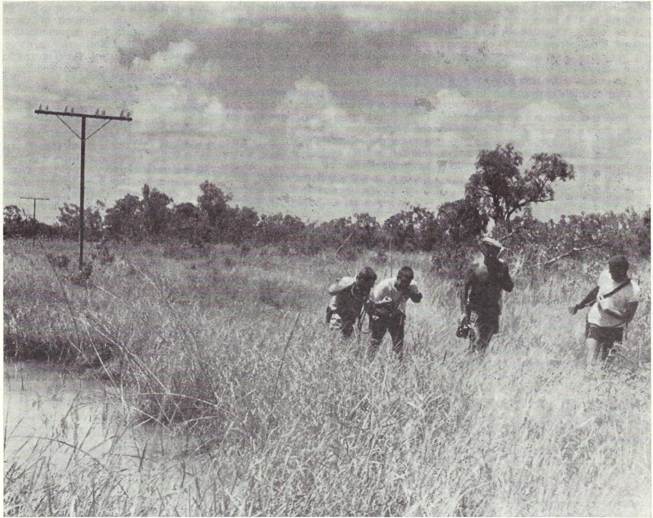
Fig. 2. — The Difficult Conditions Met by the Original Construction Teams Recur Annually. Linemen are shown erecting wires in flooded country near Larrimah in February 1966.
