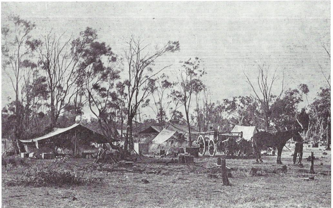
Fig. 4. — Typical Temporary Camp of a Line Construction Party.
