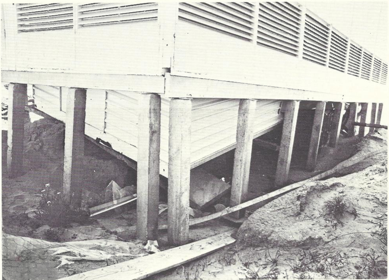
Fig. 6 — Sand Erosion at Site MP18.
