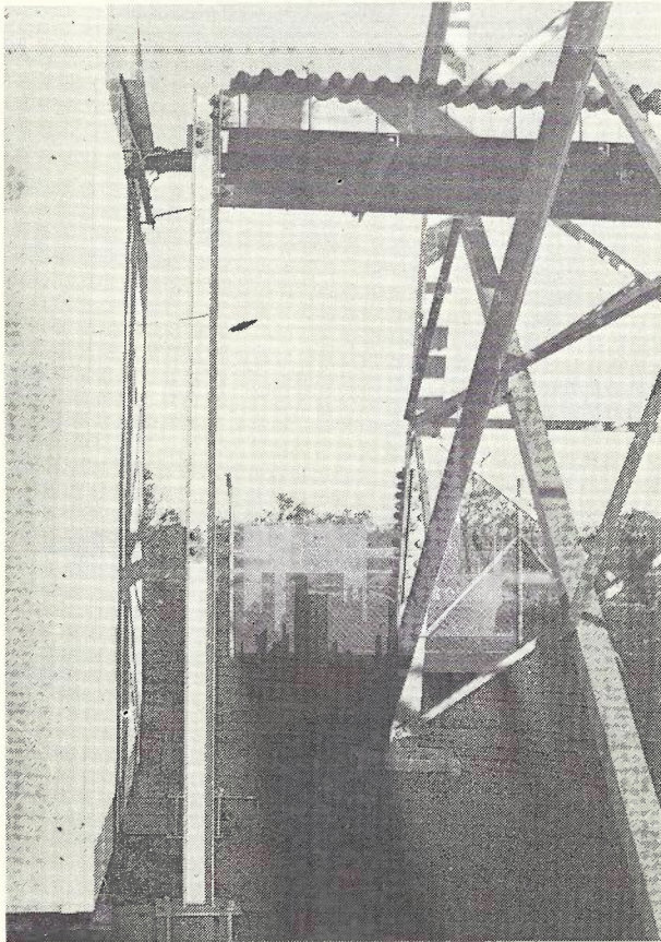
Fig. 10—Repeater Waveguide Gantry. Note Attachment to Shelter Main Members.
