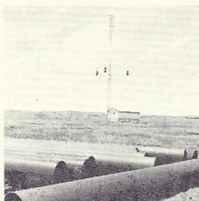
COVER RADIO REPEATER STATION
