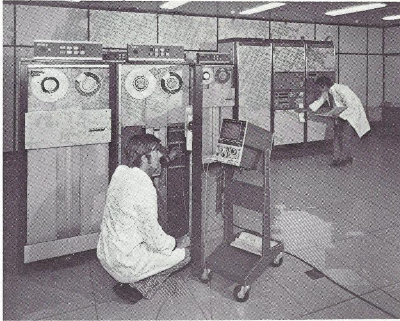
Fig. 6.—Pitt 10C Trunk — Service Control Room with Magnetic Tape Reload Cabinets (in foreground) and Service Control Racks (in Background).
