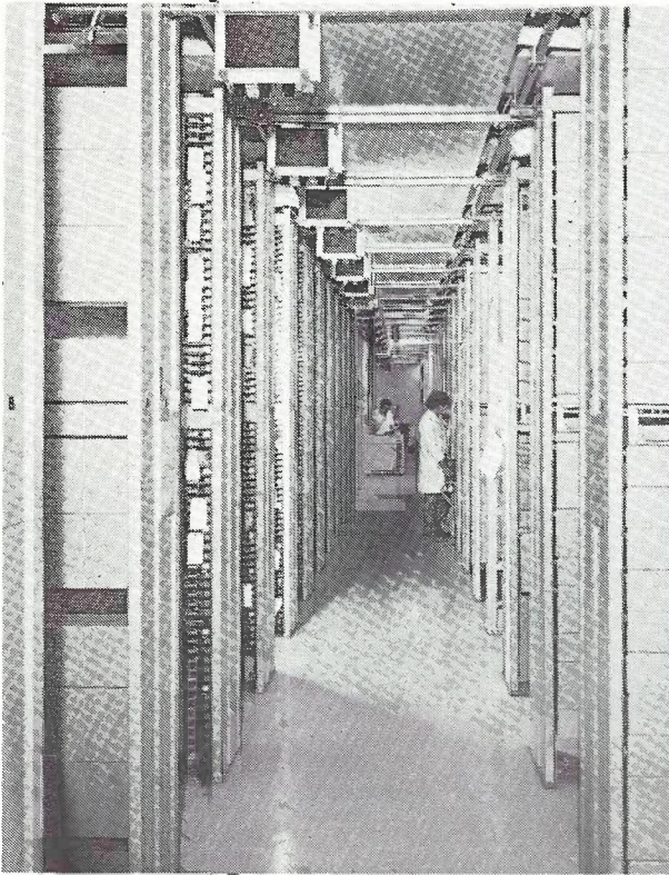
Fig. 3.—View Down Central Equipment Aisle — ARF Equipment Room — 5th Floor.
