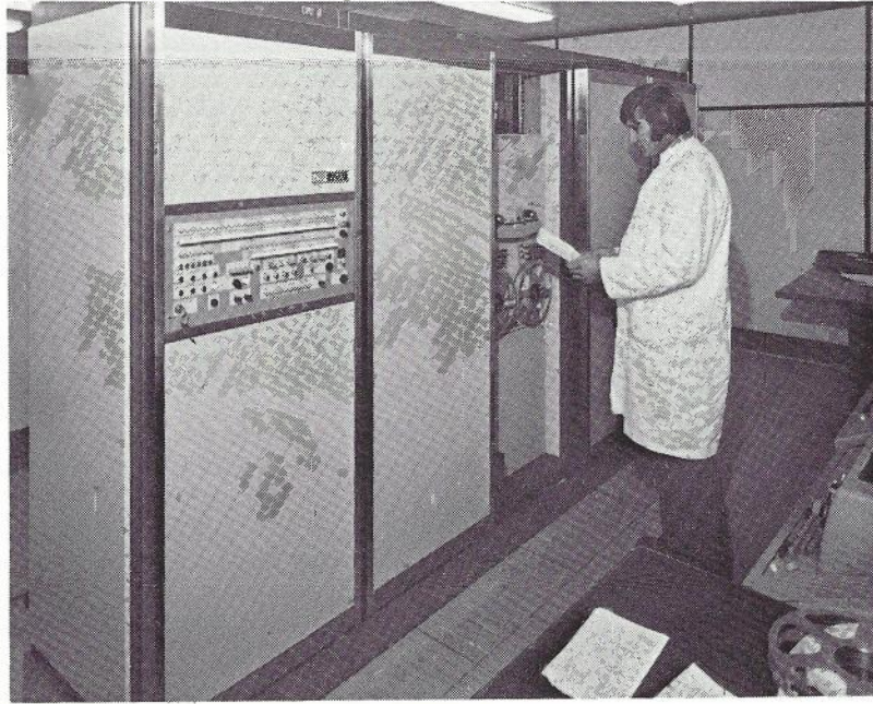
Fig. 5 — Pitt 10C Trunk — Processor Room with ITT3200 Central Processor Control Panel (left) and Paper Tape Reader.
