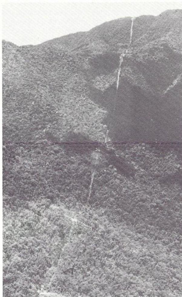
Fig. 8—Cleared Cableway Track to Top Site.
