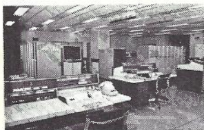
COMPUTER ROOM BRISBANE CUDN CENTRE
