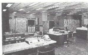
COMPUTER ROOM BRISBANE CUDN CENTRE
