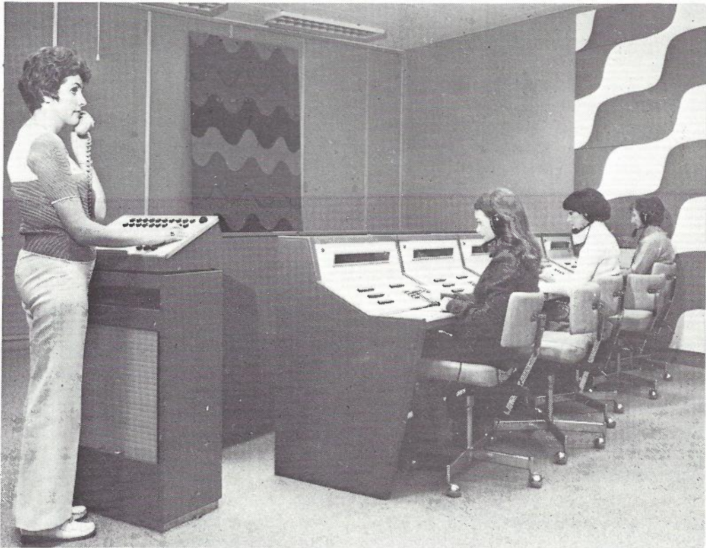
Fig. 3 — Operators' Consoles with Monitor's Post.
