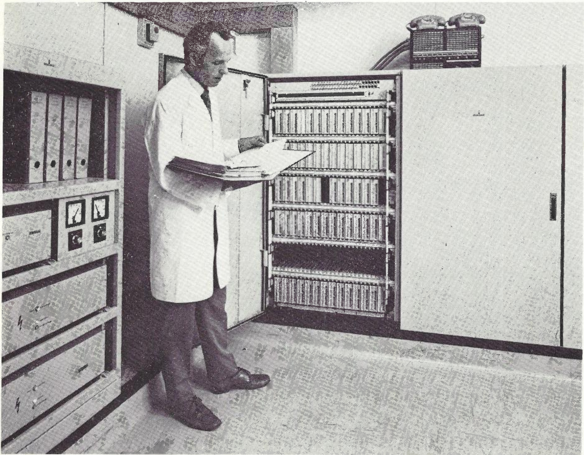
Fig. 8—Siemens ESK 60/400 PABX Robert Bosch, Clayton Victoria. Note test set rear top of cabinets. (Photograph courtesy Siemens Industries Ltd.)
