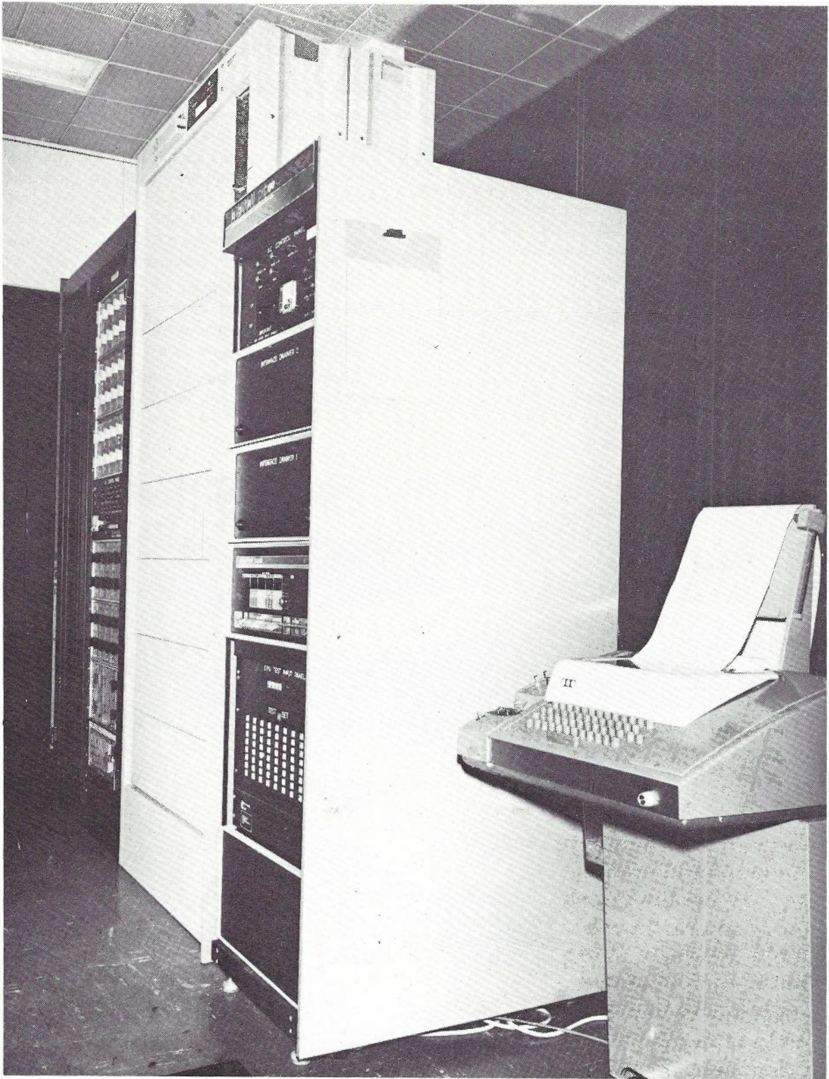
Fig. 6—Rubin "System R" ACD Equipment, NRMA, Sydney.
