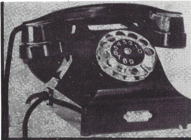
L. M. Ericsson (Sweden) really started something with this design in 1932. Many countries followed with their own versions including England and Australia, with our 300 and 400 series. Note unusual dial numbering.
