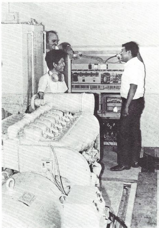
Fig. 10—Jakarta Power Plant Installation.
