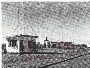
COVER BIRDSVILLE RECEIVING STATION
