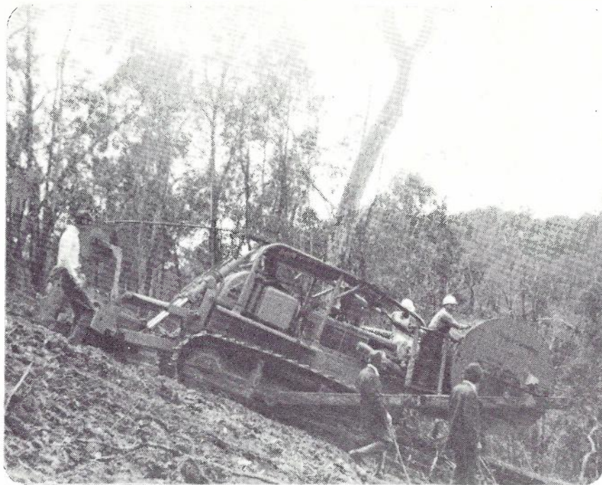
Fig. 2 — Moleplough Installing Cable.
