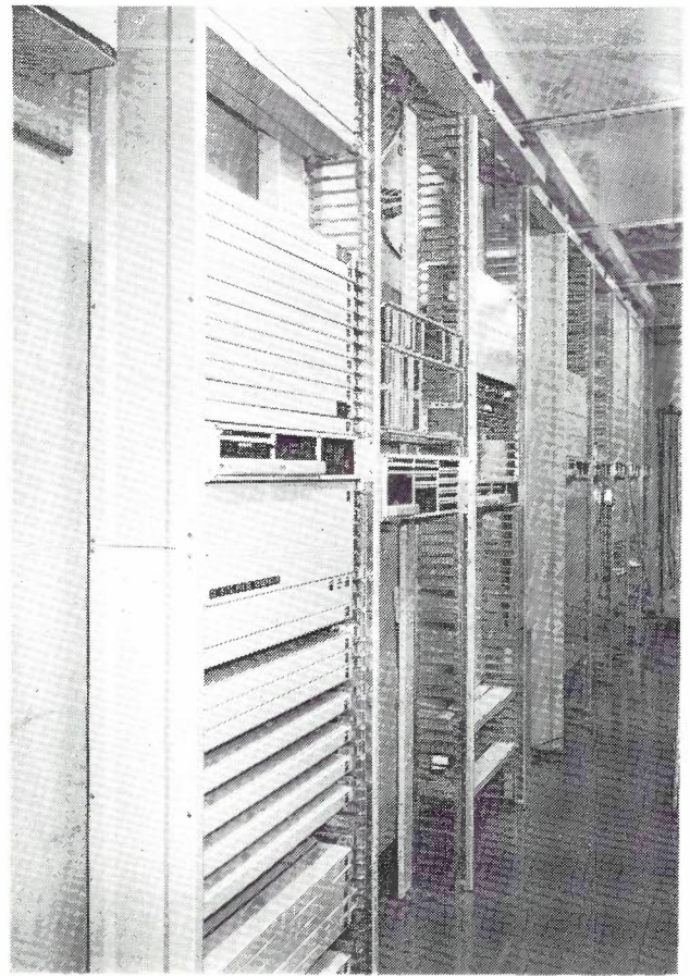
Fig. 6 — New Tariff Equipment Racks
