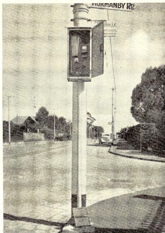
Fig. 6.—Boosted type drainage bond for electrolysis protection.
