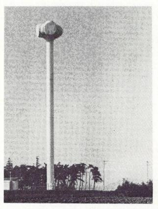
Fig. 4 — Japanese 18-20 GHz Radio Repeater
