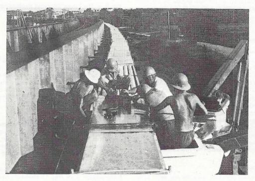
Fig. 11 - The Lids being Bolted into Position.
