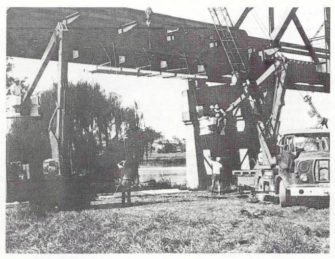
Fig. 10 — The Troughing being Lifted into Position.
