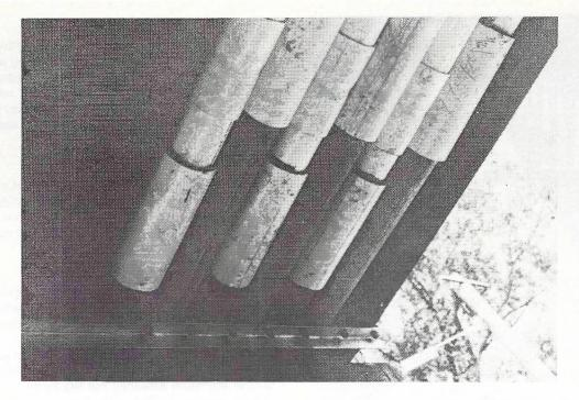
Fig. 6 — The Expansion Joints used as the Interface between the GI and PVC Conduits.
