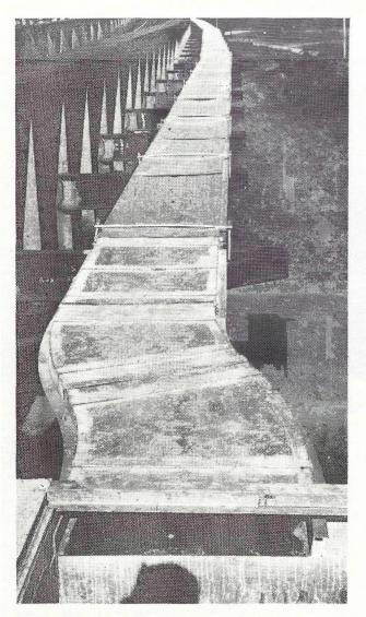
Fig. 8 — The 'S' Shaped Trough.
