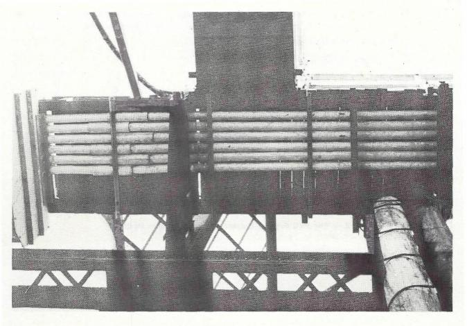
Fig. 4 — The Expansion Joints (Left of Picture).
