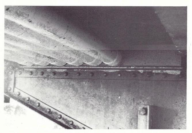
Fig. 3 — The Anchor Plate Welded to Footpath Support Bracket.
