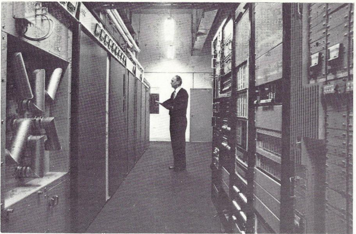
Fig. 3 — Input Equipment and Transmitter Coaxial Patch.
