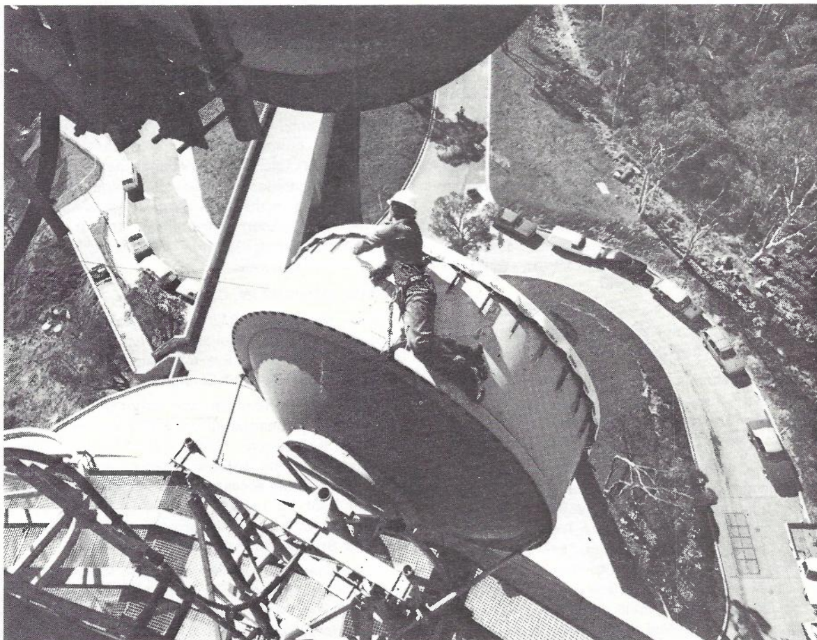
Installation of Radio Relay Dish Antenna on RT Drum
