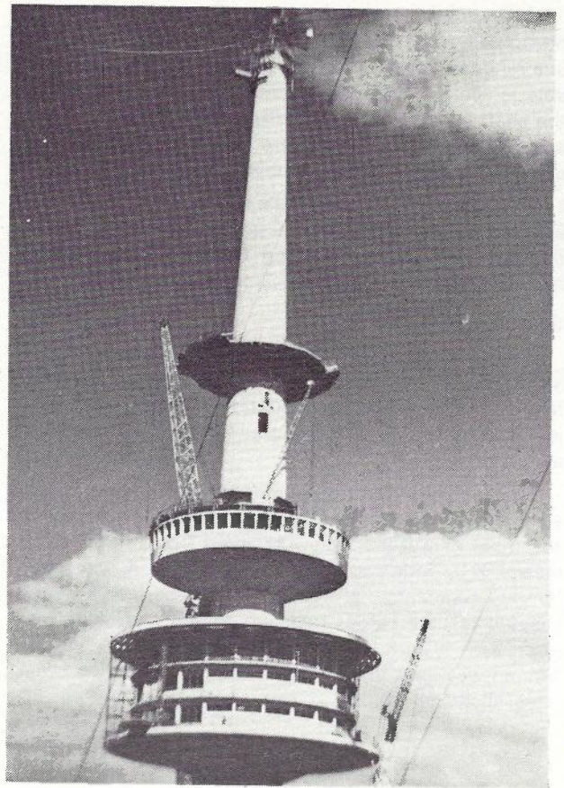
Fig. 10 — Construction with Shaft Nearing Completion and Drums Well Advanced
