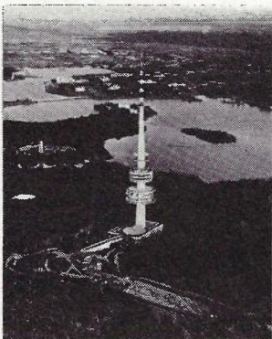
COVER: Telecommunications Tower, Canberra
