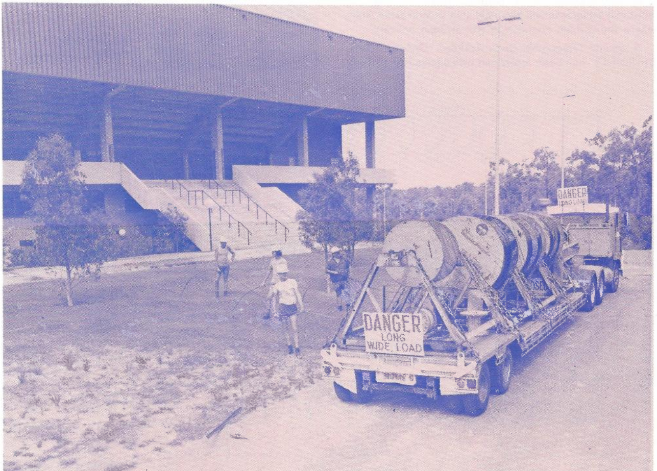
A cable hauling team from Telecom's Newstead's Line Depot in Brisbane, feed video cables into the Chandler Aquatic Centre, one of the venues on which most interest will centre during the Commonwealth Games.
