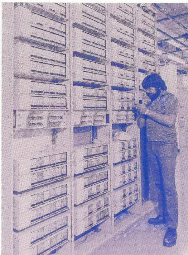
Fig. 12 — 10kHz Program Equipment Installation — Woolloongabba.
