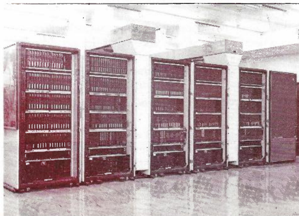
Fig. 1 — AWA —D2000 PABX/ACD Installation Ansett Melbourne.
