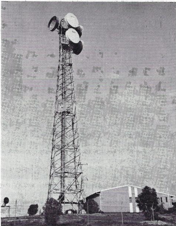
Fig. 3 — Kalgoorlie Microwave Terminal. Leonora System Antenna is in Top Left Position.
