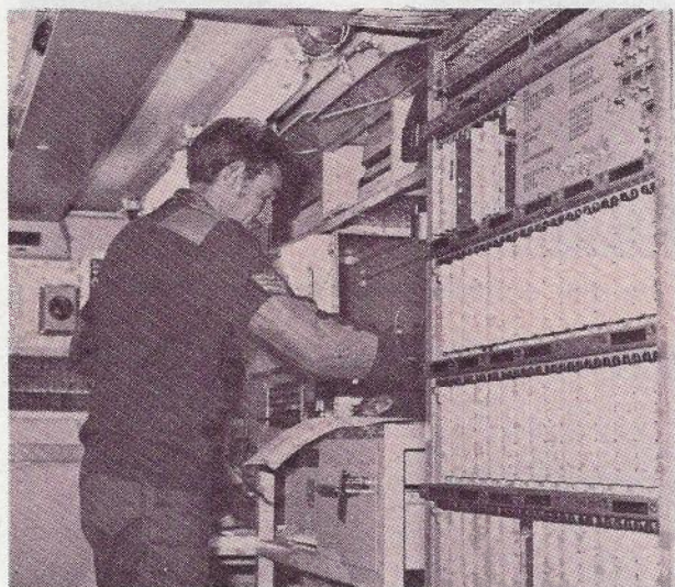
Fig. 5 — Inside the Field Automatic Telephone Switch shelter. It is an only slightly modified 150 line Australian made PABX.
