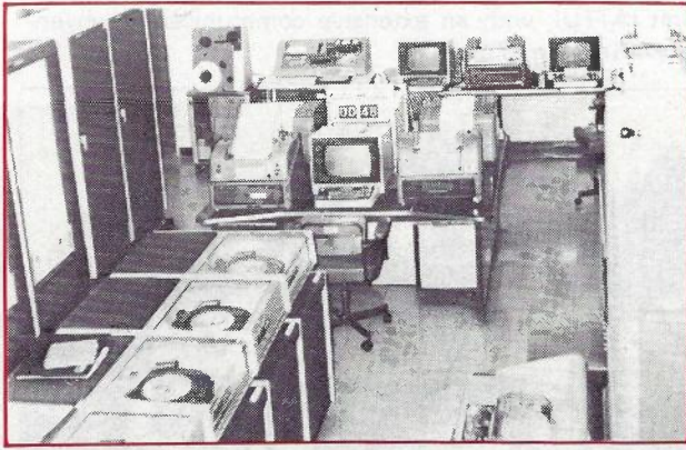
Fig. 8 — View of section of RAAF first generation automated message switching centre.
